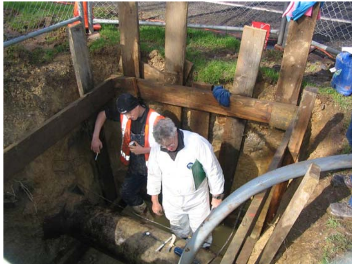
Photo 1. In-situ assessment of DN 375 AC pipeline.
