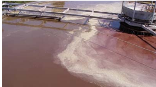
Photograph 3: Bloody wastewater in a clarifier in primary settling tank at a slaughterhouse.
