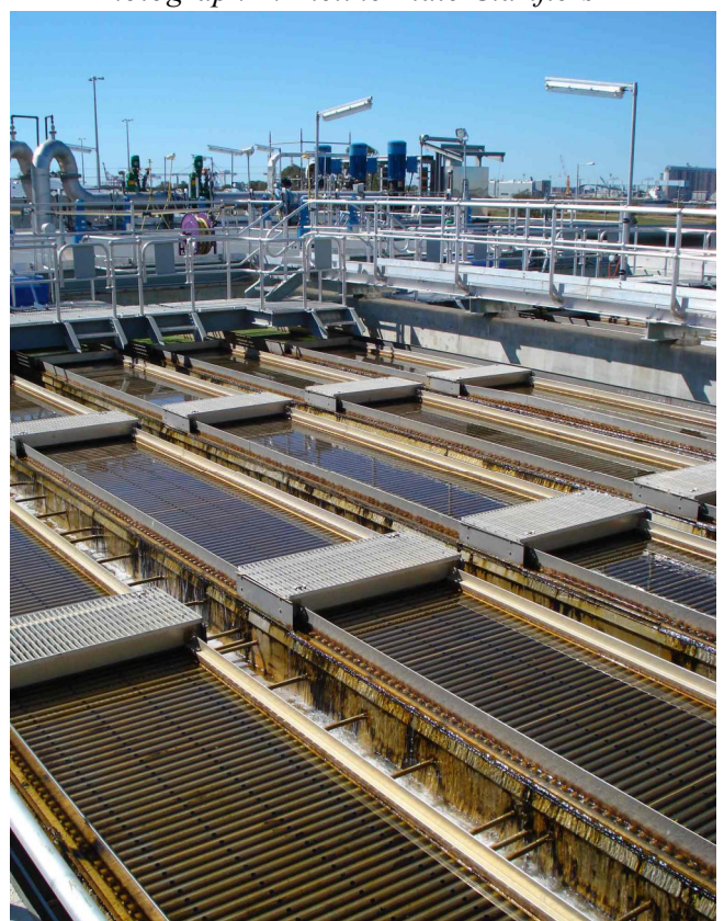
Photograph 2: Incline Plate Clarifiers
