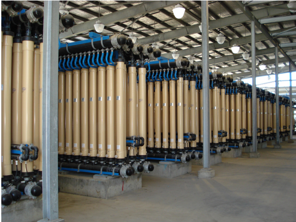
Photograph 4: Microfiltration system.
