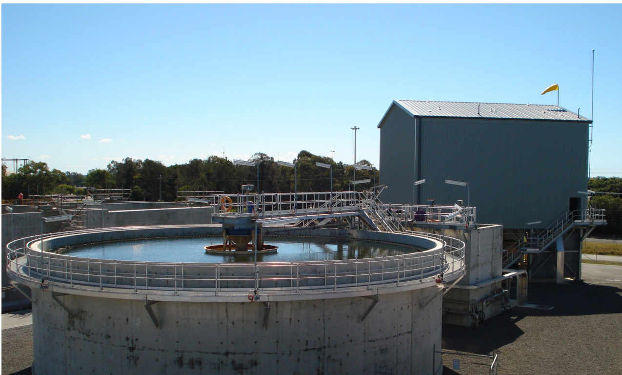
Photograph 3: Thickener clarifier and dewatering building
