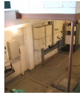
Figure 15 Auburn PS Building
