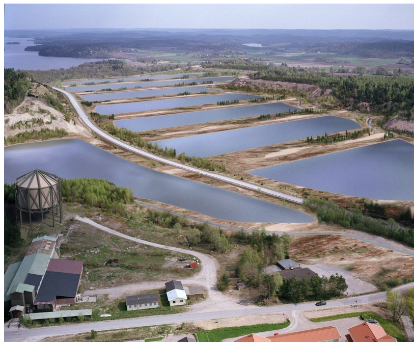
Figure 1 A photo visualisation of the planned MAR plant at Lake Mjörn in Sweden.
