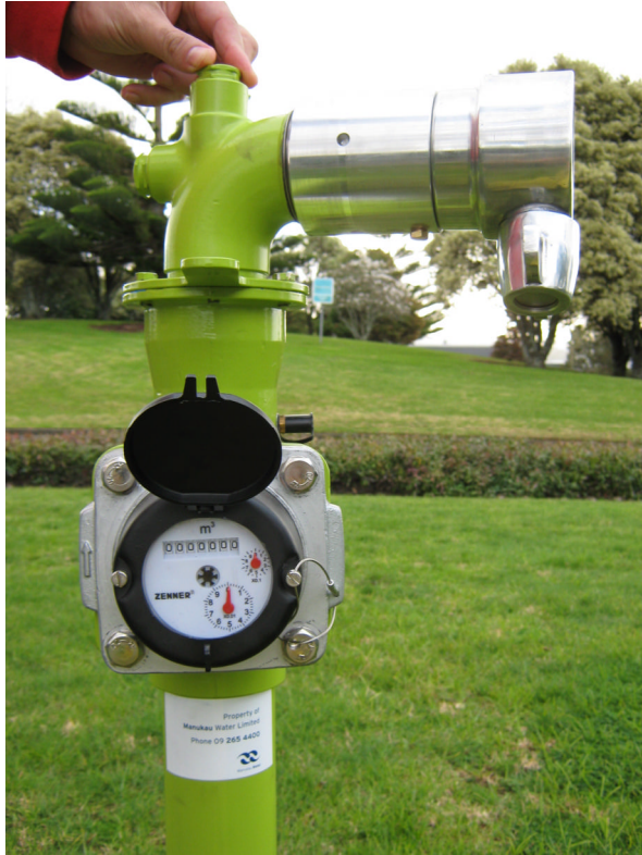
Figure 6: Standard Standpipe for Hydrant Flushing
