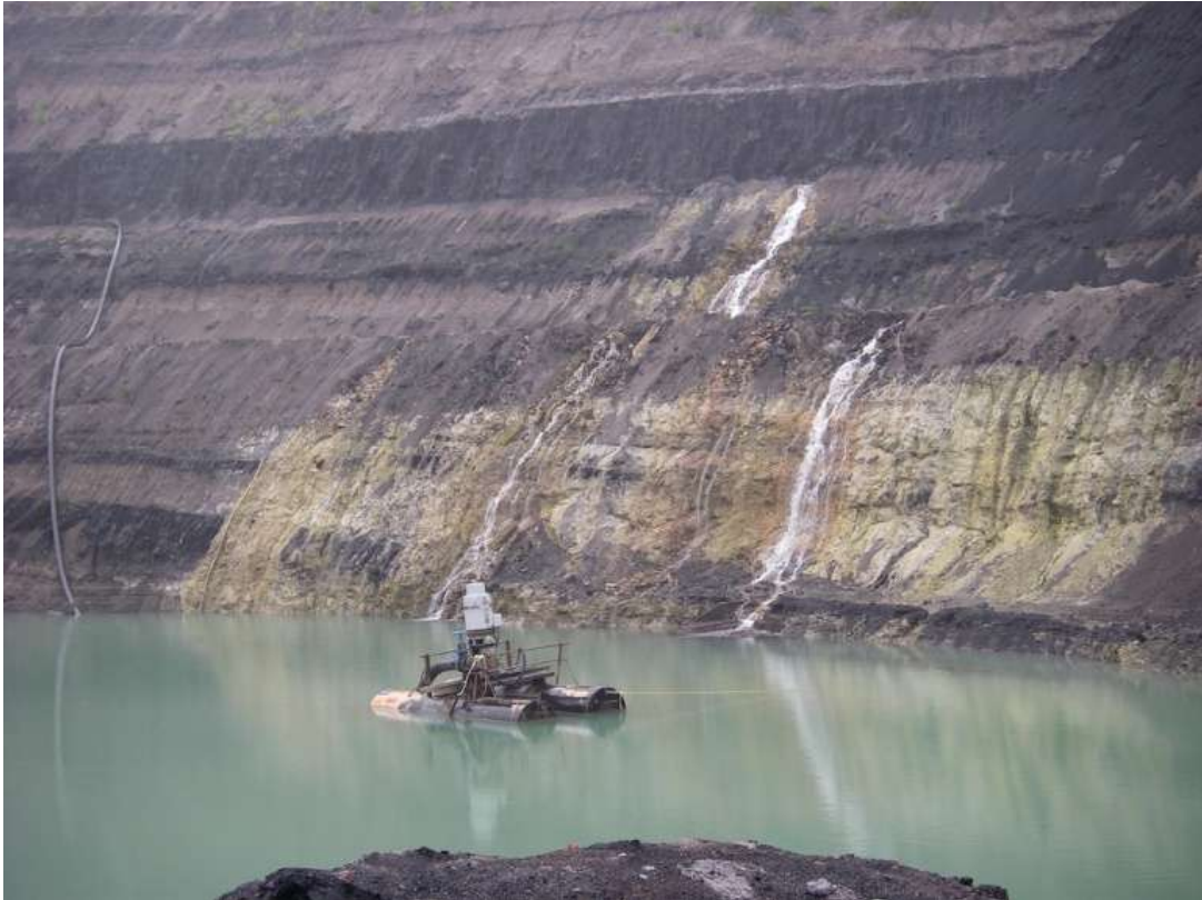
Figure 3 - A submersible pump supported by a flotation raft in the Awaroa 4 pit sump
