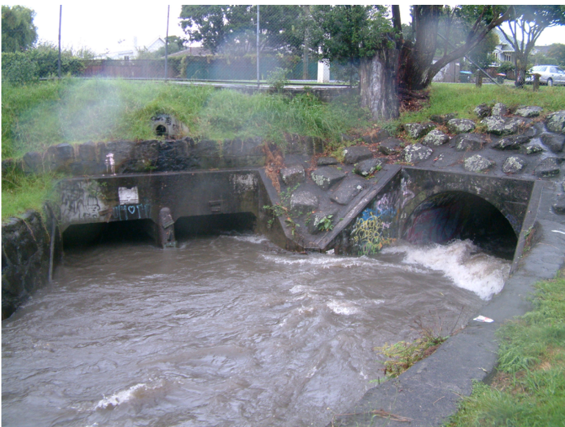
Figure 2: Bollard Avenue Culverts
