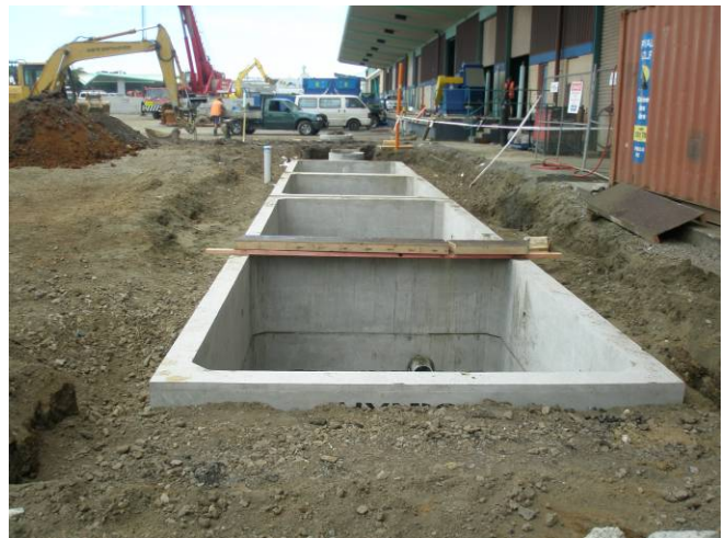
Photographs 4 & 5: Installation of sand/peat filter tanks in Area B & Sand/peat filter tanks in Area C after backfilling.
