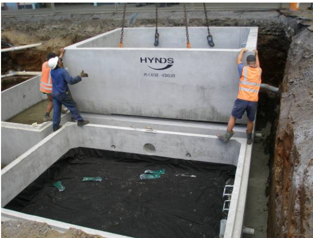
Photographs 4 & 5: Installation of sand/peat filter tanks in Area B & Sand/peat filter tanks in Area C after backfilling.
