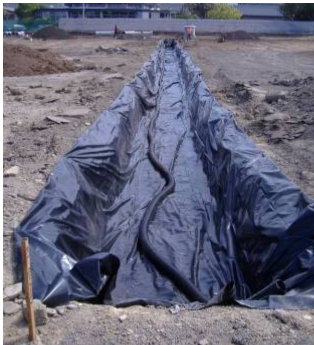
Photograph 2: Excavated rain garden showing underdrain and impermeable liner installed.
