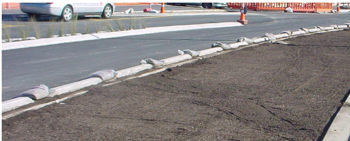
Photograph 1: Constructed rain garden showing sand bags blocking inlets for protection.
