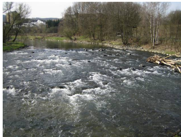
Photographs 6 & 7: Rockfill ramp with perturbation boulders ( S \approx 1:35 ) in Husten, Ruhr River, Germany during extreme low and mean flow conditions
