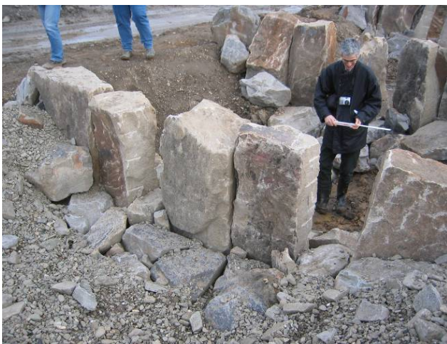
Photograph 10: Pool & boulder-type fish pass Harkortsee, Ruhr River, Germany during construction
