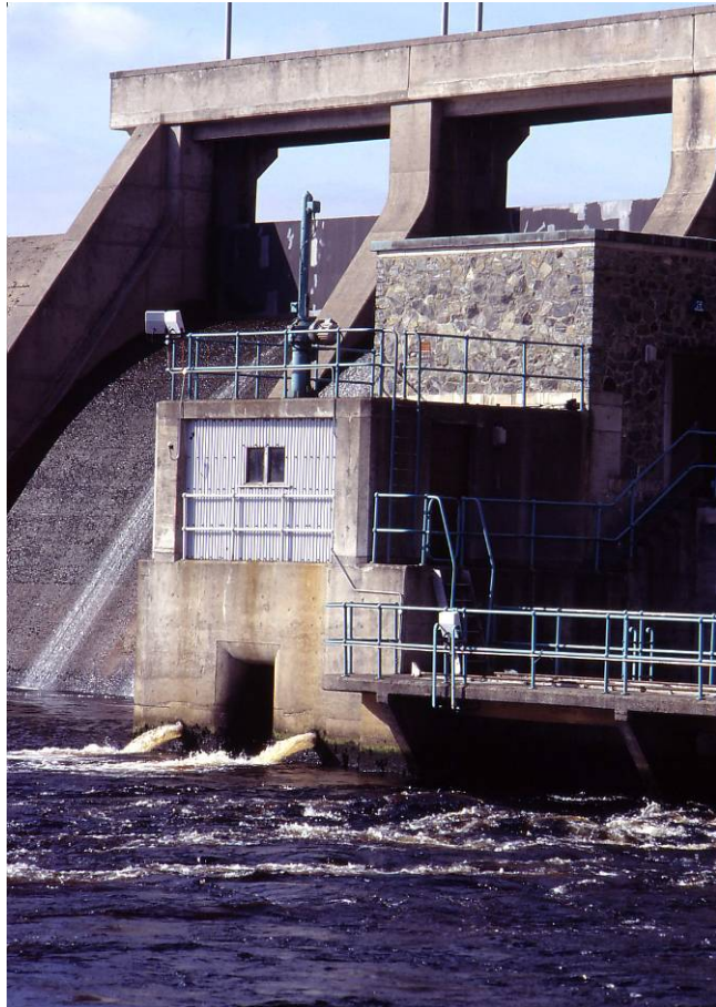
Photograph 3: Fish lock entrance adjacent to the draft tube outlet of a hydropower plant and attraction flow entering parallel to the main flow. Lairg Dam, Scotland (photo: Scottish Hydro)
