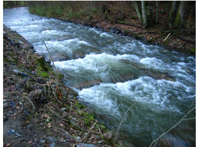
Photograph 9: Combined rock-ramp fishway in Olsberg, Ruhr River, Germany during high flow conditions
