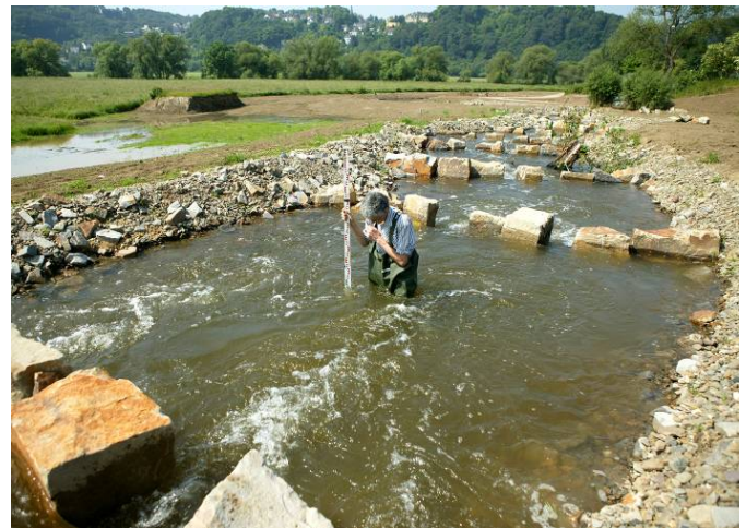
Photograph 11: Pool & boulder-type fish pass Harkortsee, Ruhr River, Germany during test runs
