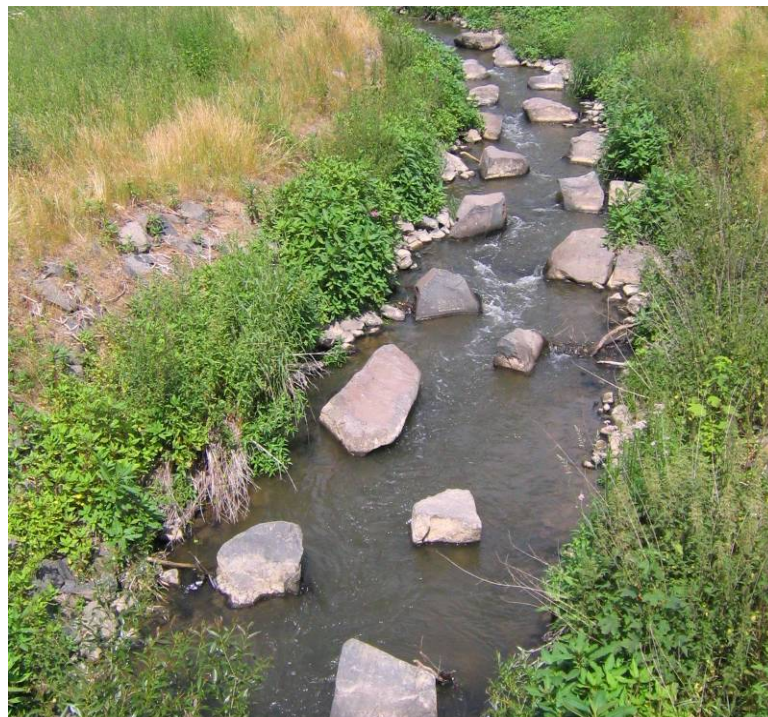
Photograph 12: Nature-like bypass channel Hadamar, Elbbach, Germany with perturbation boulders
