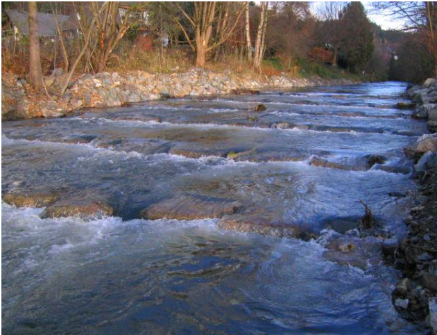
Photograph 8: Pool & boulder-type ramp in Olsberg, Ruhr River, Germany during mean flow conditions
