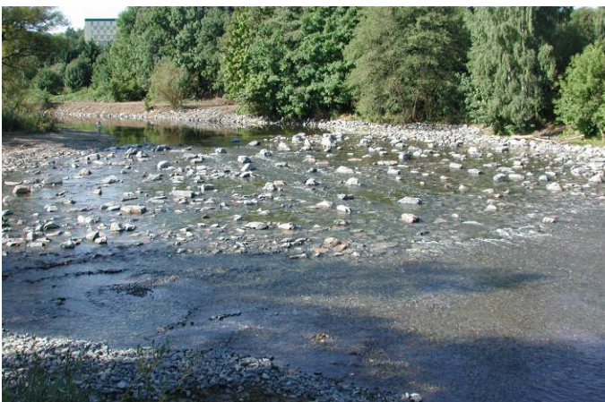
Photographs 6 & 7: Rockfill ramp with perturbation boulders ( S \approx 1:35 ) in Husten, Ruhr River, Germany during extreme low and mean flow conditions
