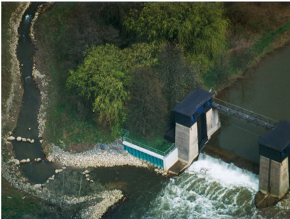
Photograph 4: Entrance of the fishway/bypass channel adjacent to the stilling basin of Beckinghausen Weir, Lippe River, Germany (photo: Lippeverband)
