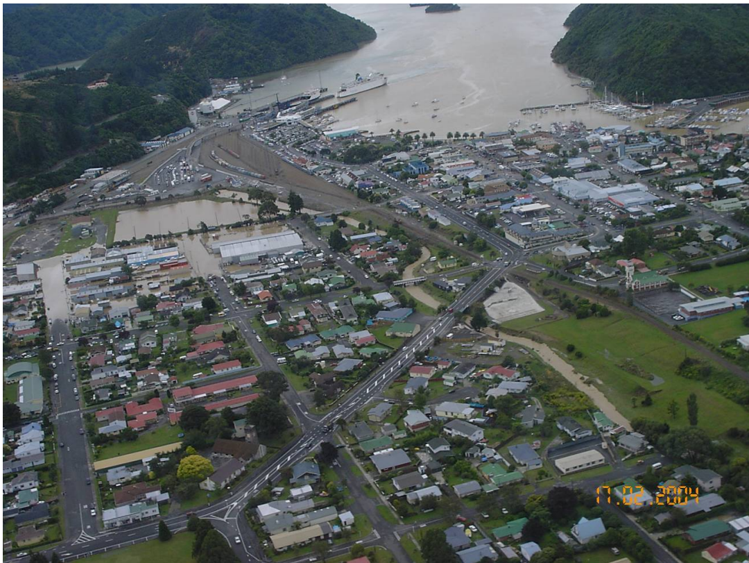
Picton February 2004, Industrial area flooded due to inadequate size of culvert under wharves
