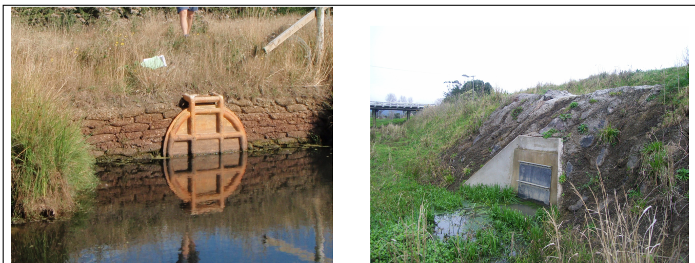
Figure 1: Pin-hinged circular (left) and flexible (right) flap gates
