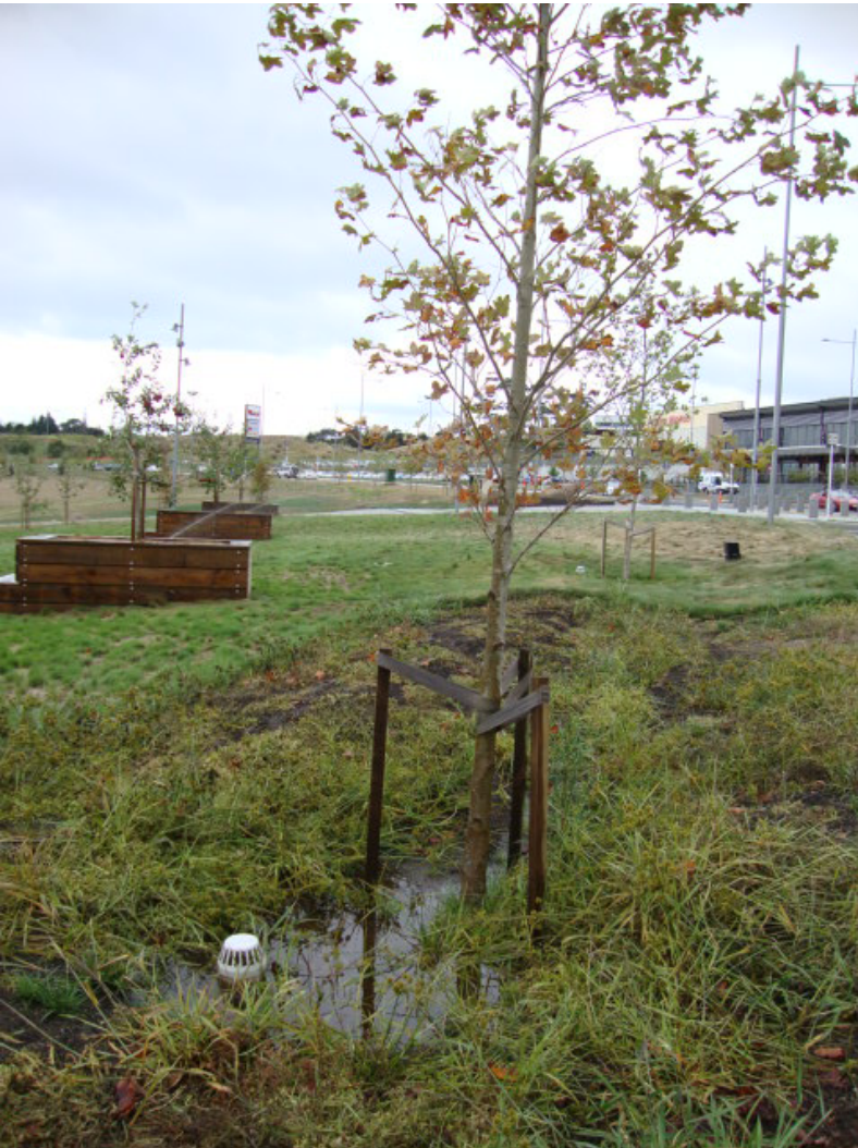
Photograph 10: Damage from excessive surface water flow during construction. Filtercloth protecting tree pit medium exposed. Park slope eroded before grass was established.
