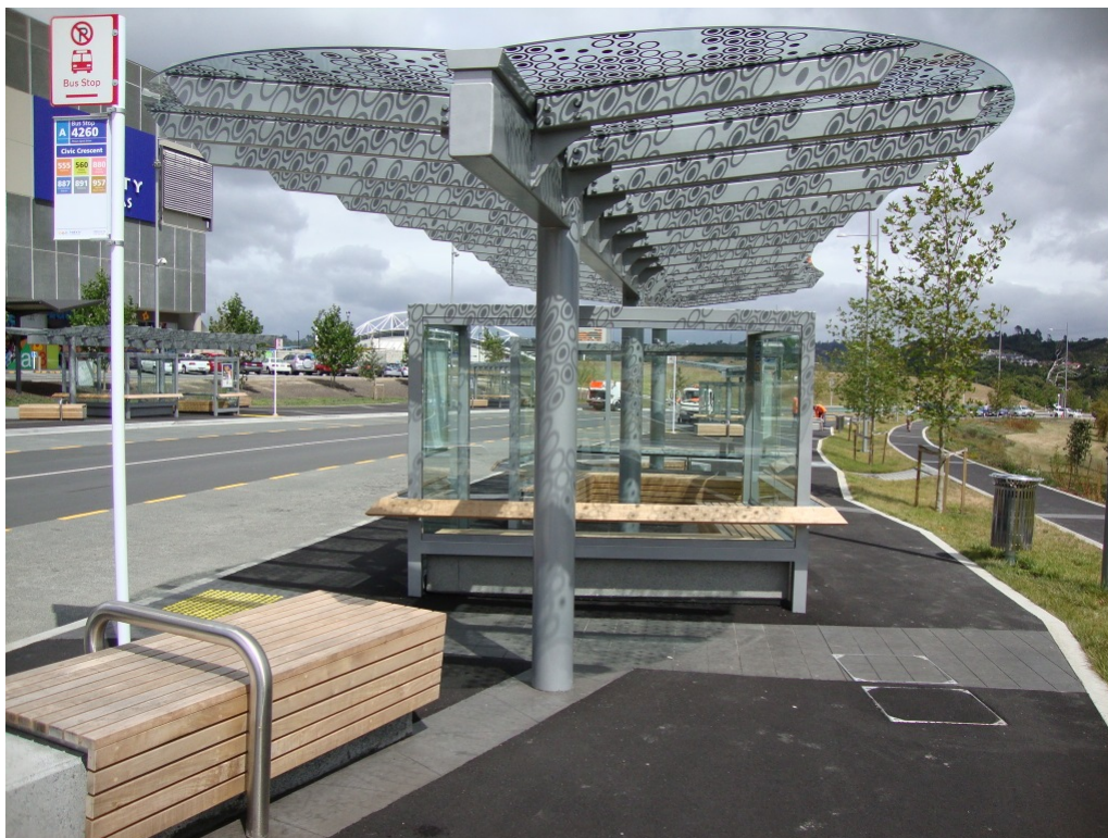
Photograph 2: Bioretention swale with tree pits between cycle path and bus station.
