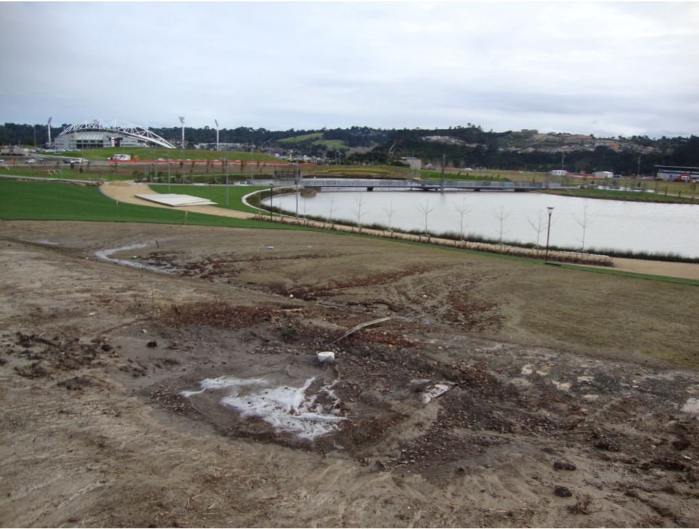
Photograph 10: Damage from excessive surface water flow during construction. Filtercloth protecting tree pit medium exposed. Park slope eroded before grass was established.
