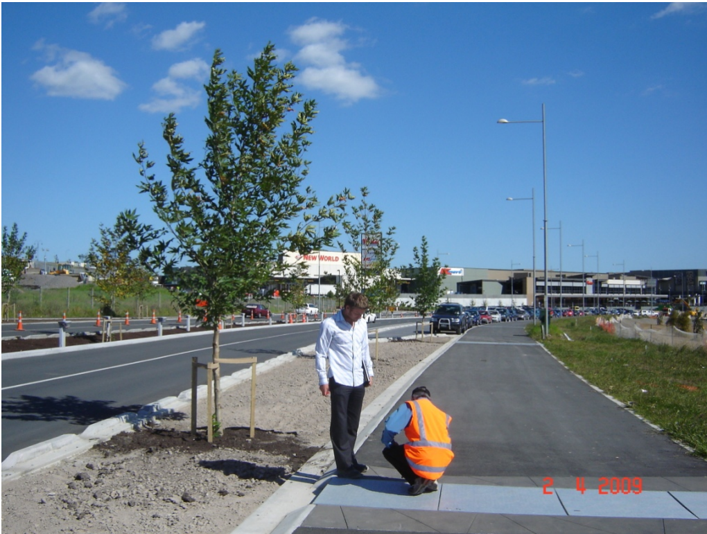
Photo 5: Cycle path at east end.
