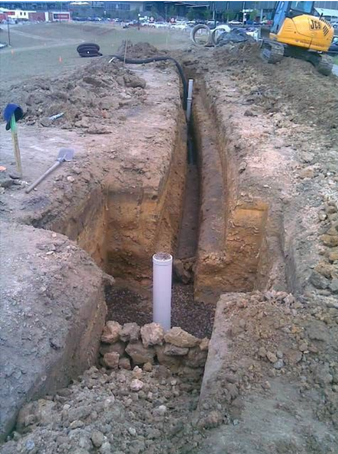
Photo 7,8,9: Bioretention tree pits during construction.
