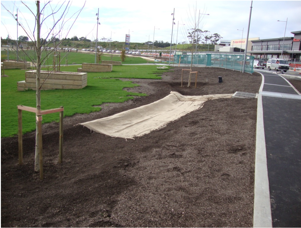
Photograph 12: Forming swale to tree pits.
