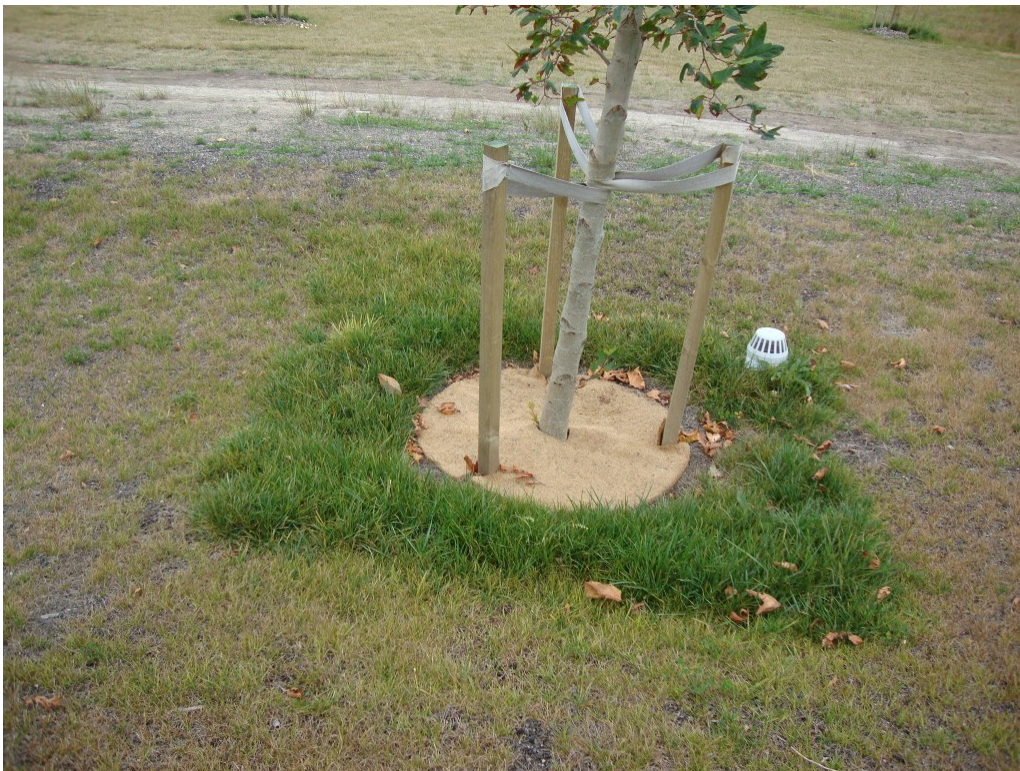
Photograph 13: Tree pits grass established. Fibre circle weed suppression. Overflow pipe inlet.
