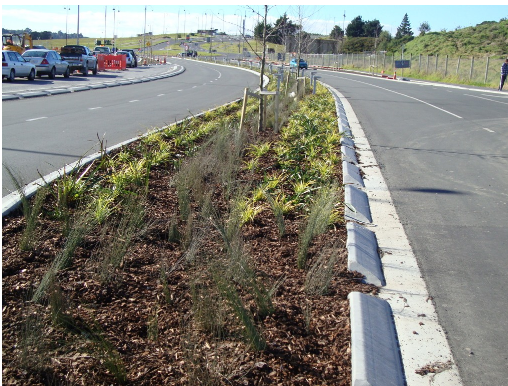
Photograph 1: Median rain garden with tree pits
