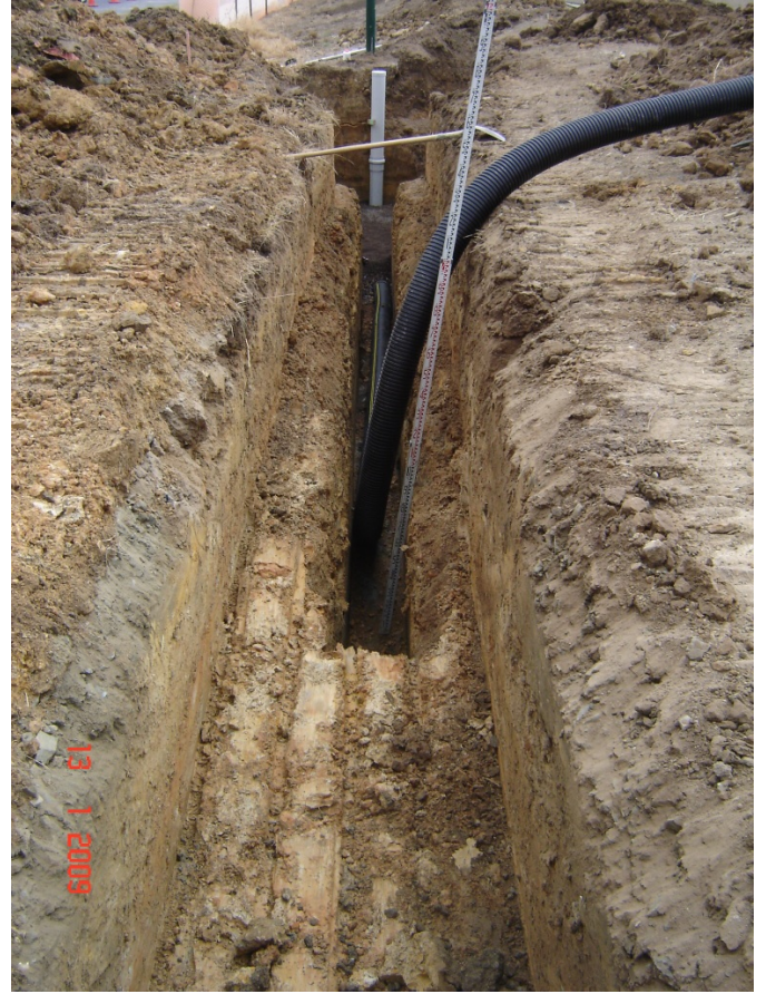
Photo 7,8,9: Bioretention tree pits during construction.
