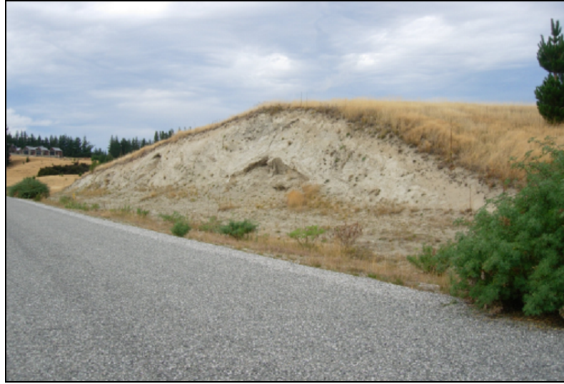
Figure 5: Large Cut adjacent to Kirimoko Crescent
