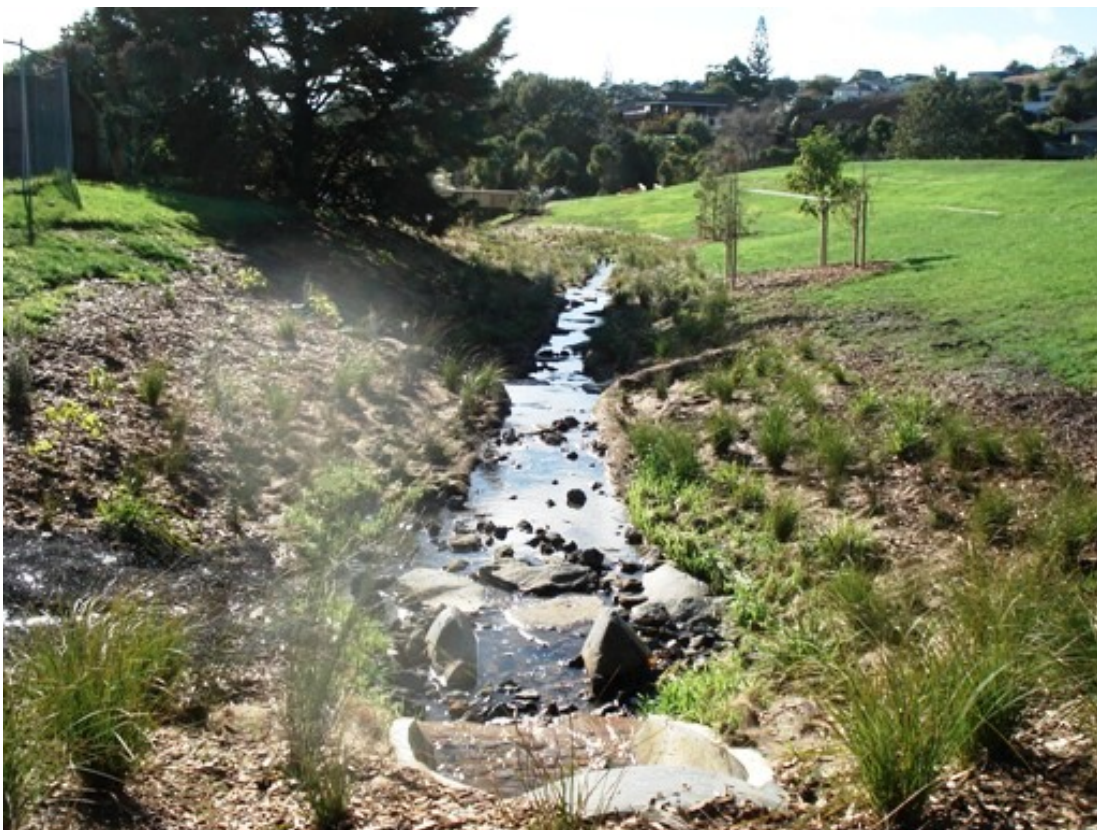
Figure 9: Northern Channel after restoration
