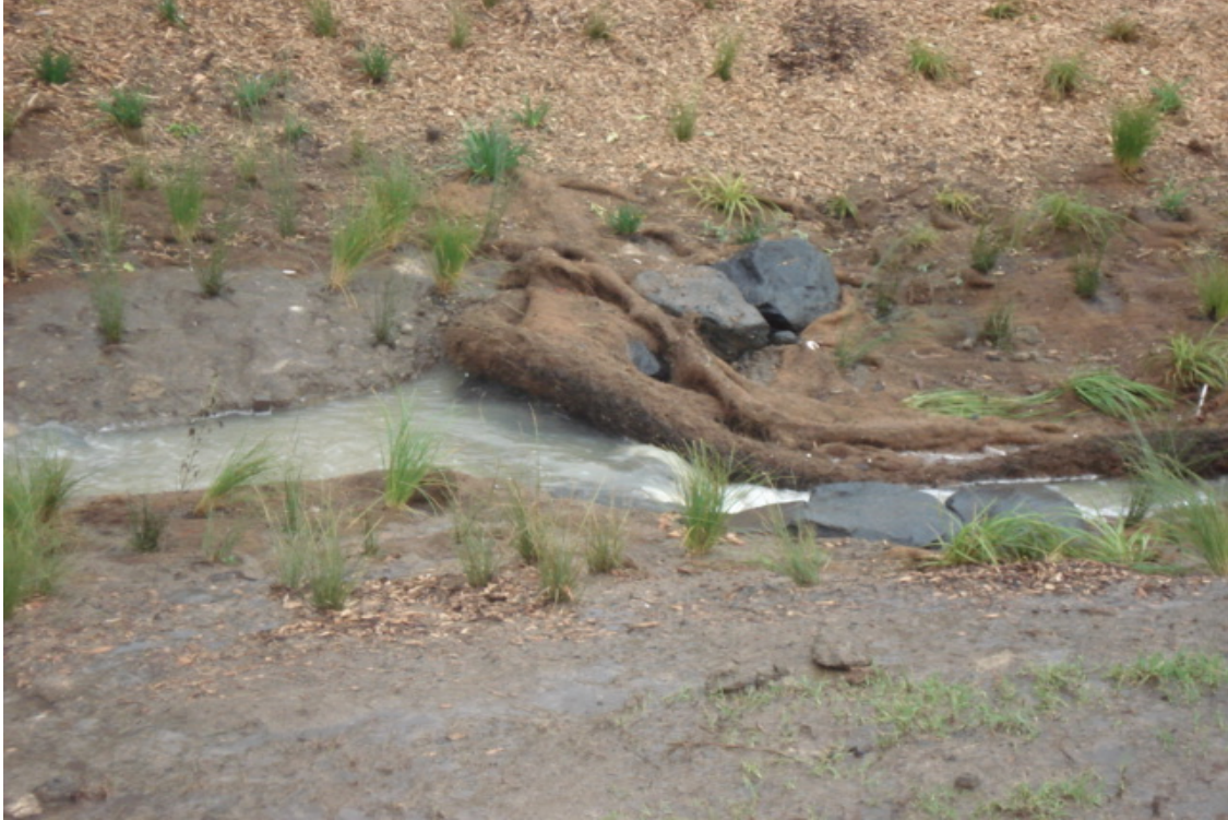
Figure 15: Coir fascines washed away during heavy rainfall
