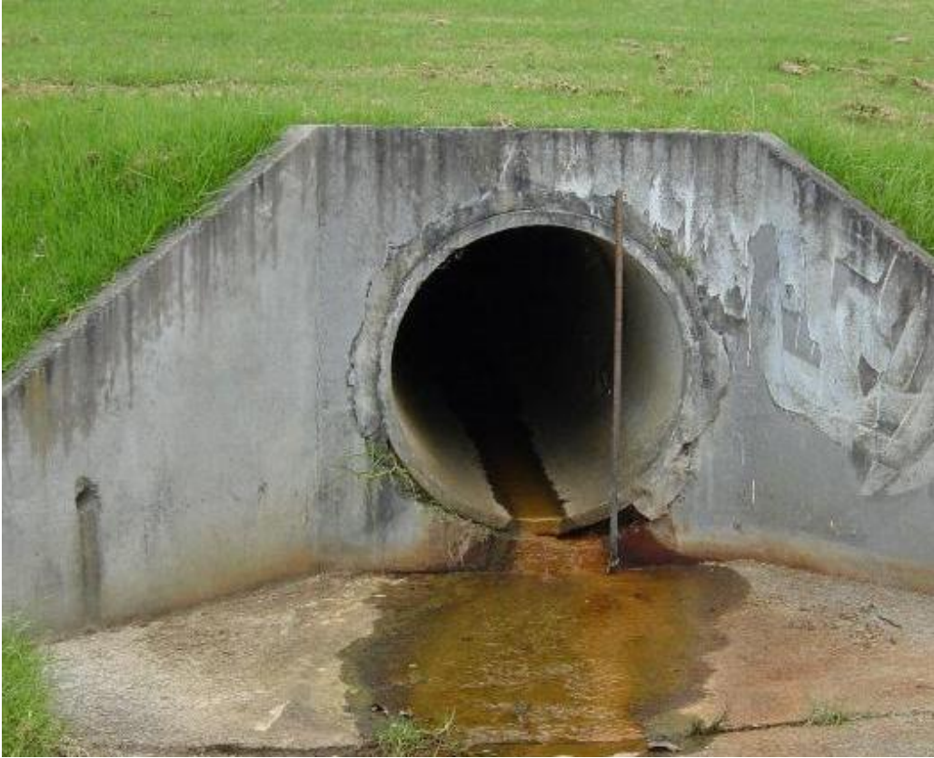
Figure 3: Northern inlet before restoration
