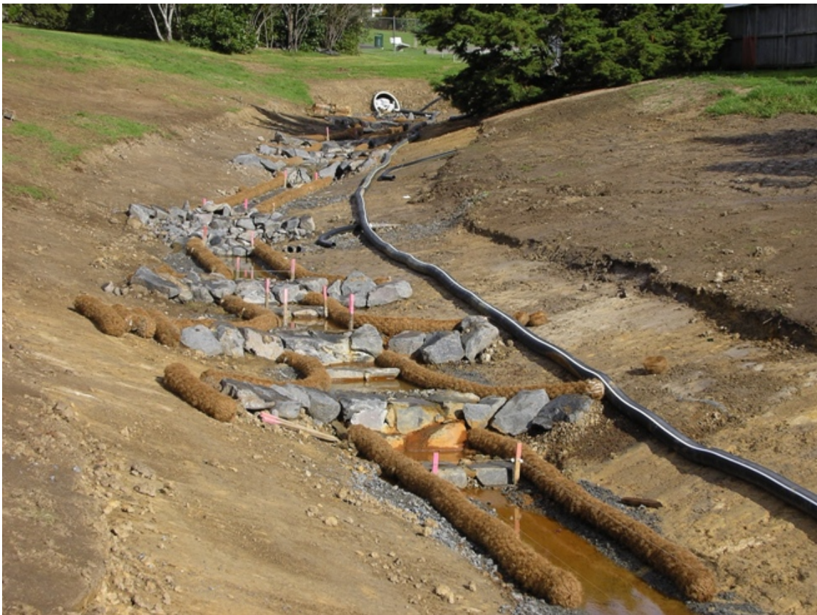
Figure 14: Stream constructed with string lines
