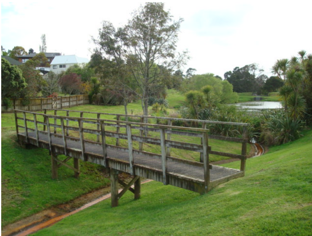
Figure 7: Existing bridge before restoration
