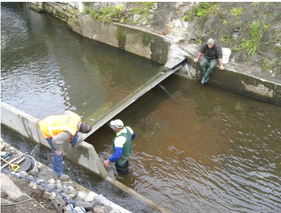
Photograph 7: Obermeyer weir being installed, July 2009
