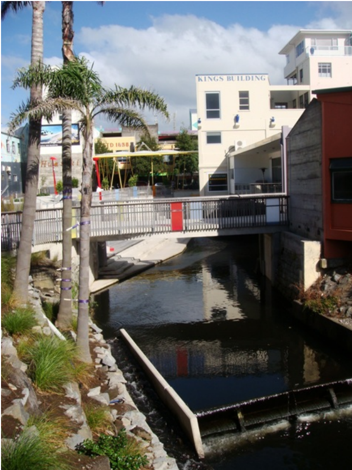
Photograph 8: Weir, fish pass, bridge, landing and plaza, March 2010
