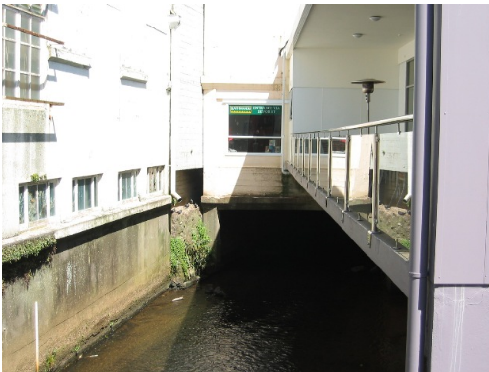
Photograph 1: Huatoki Stream looking upstream, building to be demolished on right, November 2005
