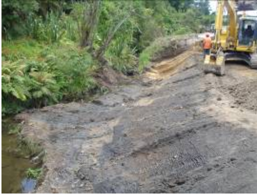
Figure 21: Berm removal
