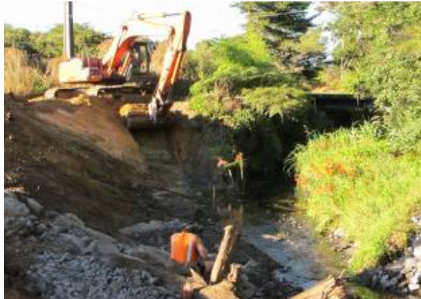
Figure 10: Rock vane under construction
