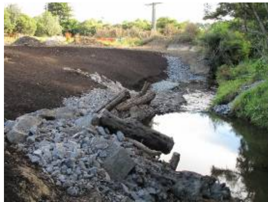
Figure 13: Rock vane completed
