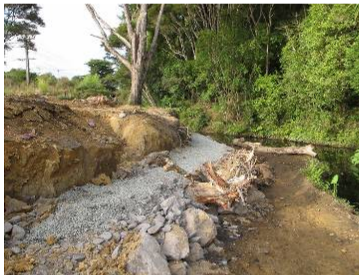
Figure 17: Rock toe with root wads
