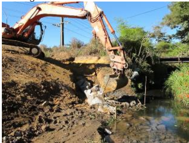
Figure 11: Rock vane under construction
