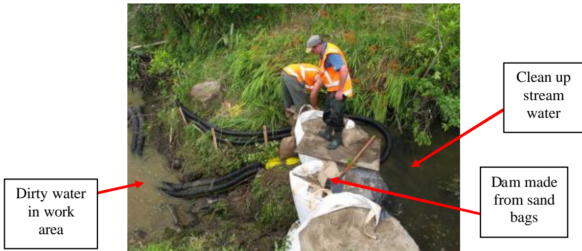
Figure 19: Damming and diverting
