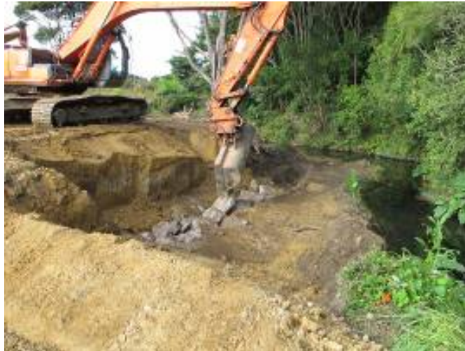
Figure 16: Rock toe under construction
