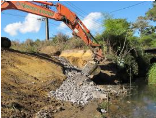
Figure 12: Placing rock
