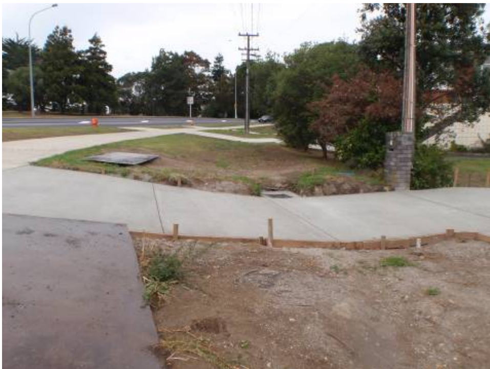
Photograph 5: An Example Of Mitigation Works To Retain Overland Flow in The Road Reserve
