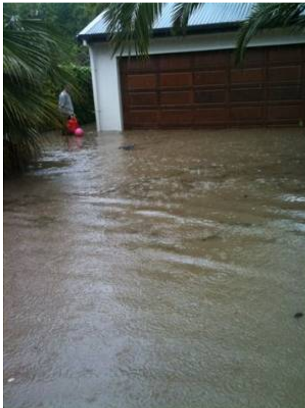
Photograph 3: Overland Flow Obstructed By Restrictive Fence behind the Garage Resulting in the Flooding of the Garage and Habitable Floors
