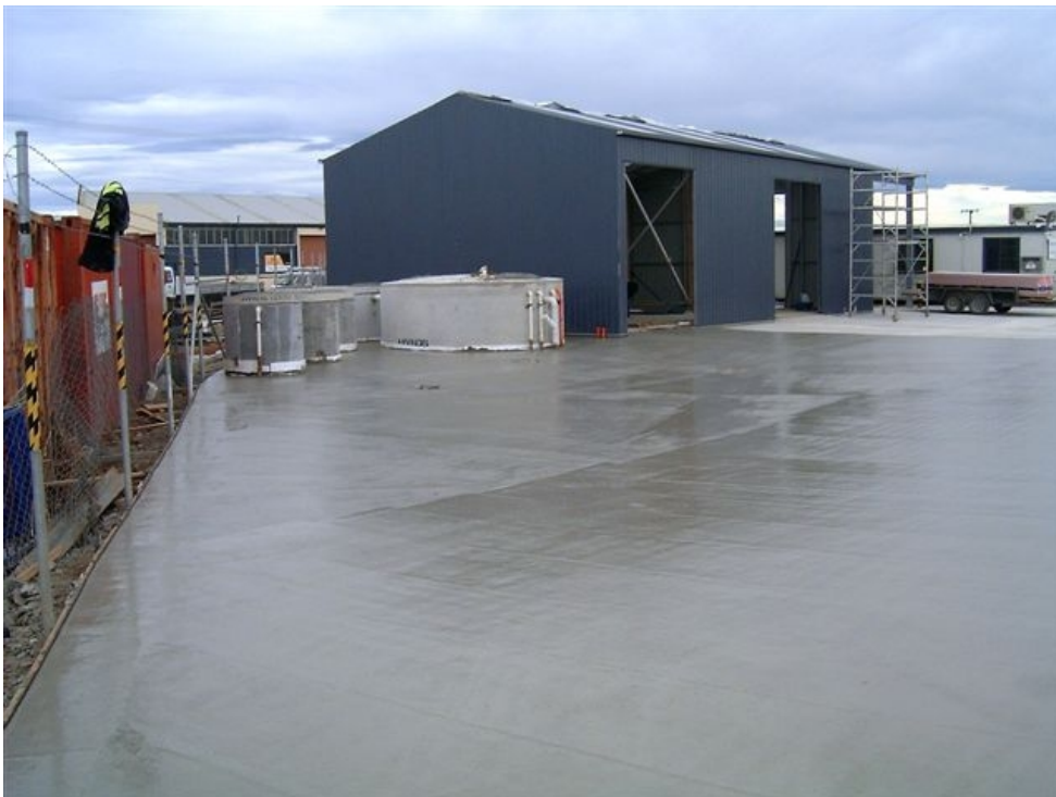
Figure 9: Treatment train in place, plumbed in, and concrete apron completed
