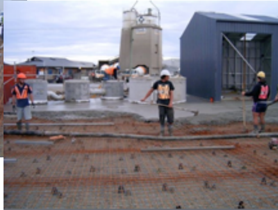
Figure 9: The treatment train laid out from left (Unit 2, 3, 4, & 6 visible)
