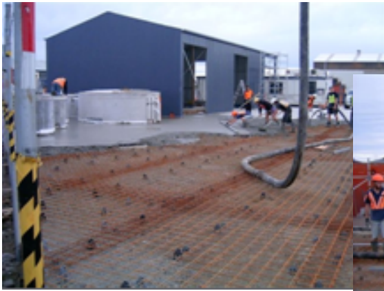
Figure 8: Laying the concrete skirt about the treatment train
