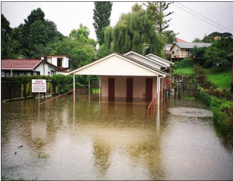
Figure 5: Example of a flooded house
