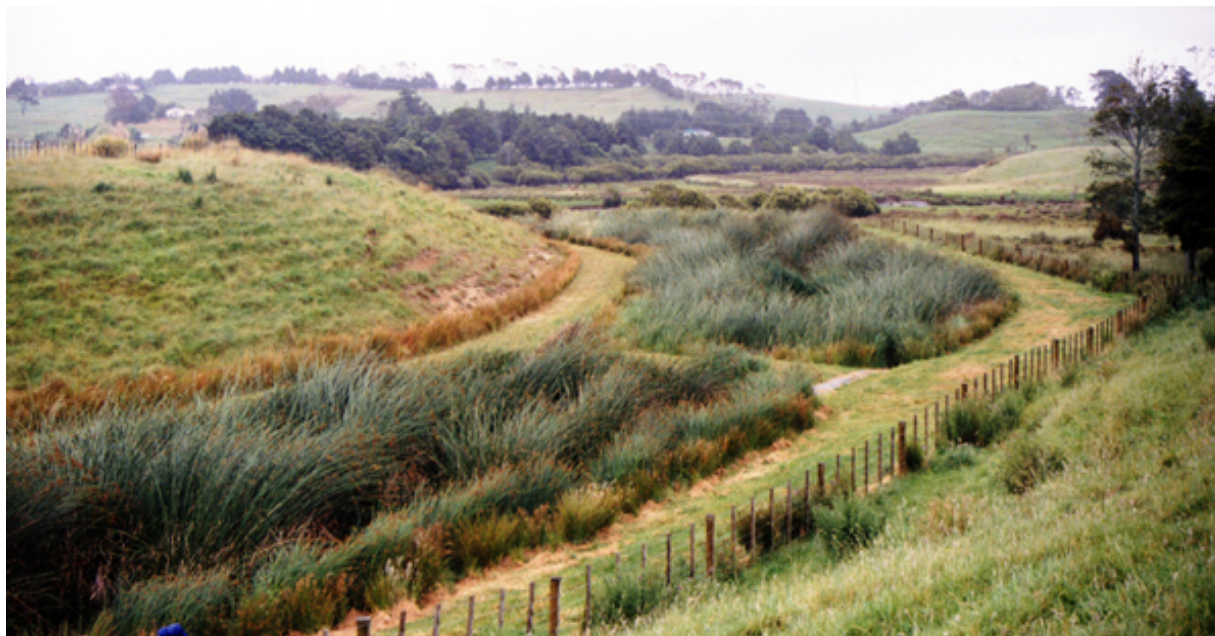
Photo 3. Surface-flow constructed wetland treating waste stabilisation pond effluents. Main species are Schoenoplectus californicus in deeper areas, with S. tabernaemontani and Bolboschoenus fluviatilis on the shallower edges.
