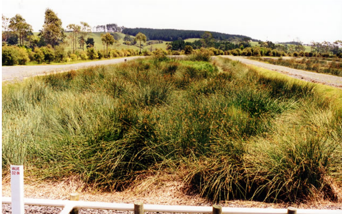
Photo 1: A well maintained surface-flow treatment wetland. The sedge Schoenoplectus tabernaemontani is the dominant species visible in the foreground
