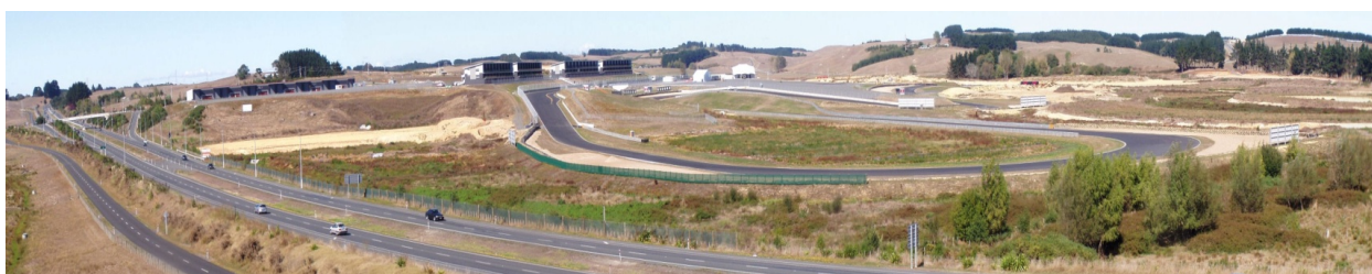
Photograph 2: During construction, showing extensive modifications of Motorsport catchment.
