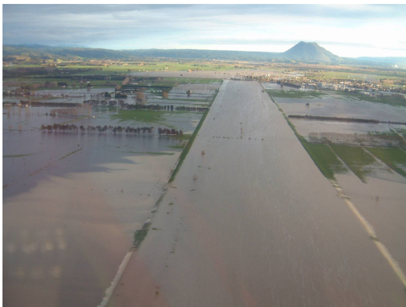
Photograph 2: Reids Floodway looking south on Sunday 19 th July with extensive overtopping both sides
