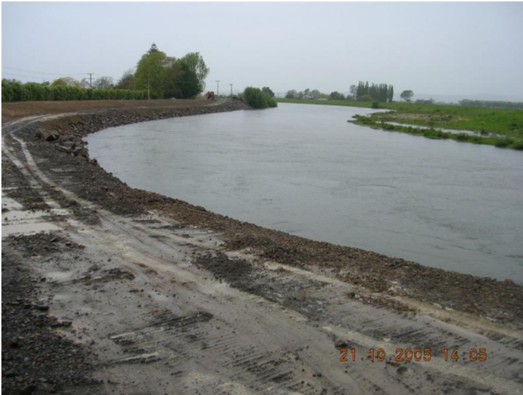
Photograph 3: Reconstruction of river bank protection works at Laws bend following 2004
