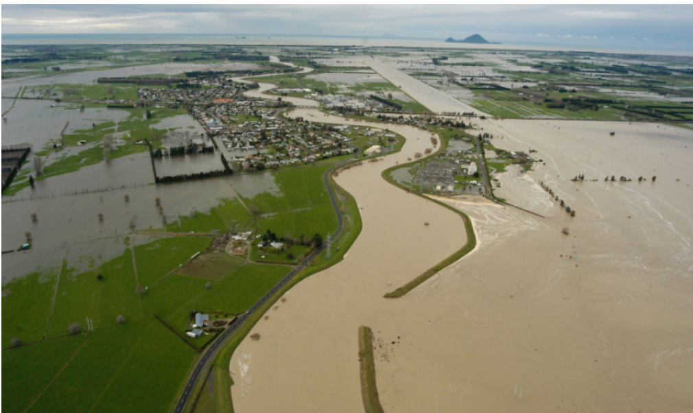
Photograph 1: Flooding in Edgecumbe and on the Rangitaiki Plains following the stopbank breach (foreground) at Sullivan's Farm
