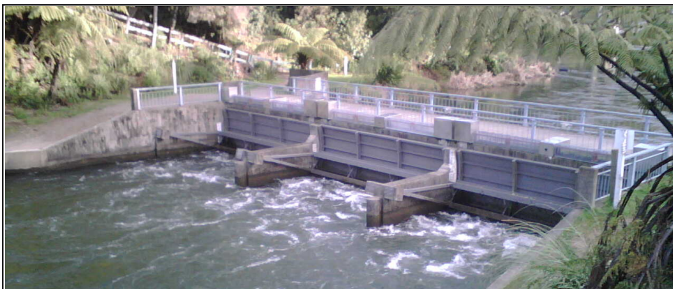
Photograph 1: Okere Gates Structure
