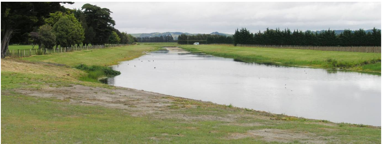
Photograph 1: Downstream end of drain, approaching pump station, looking west up the drain
