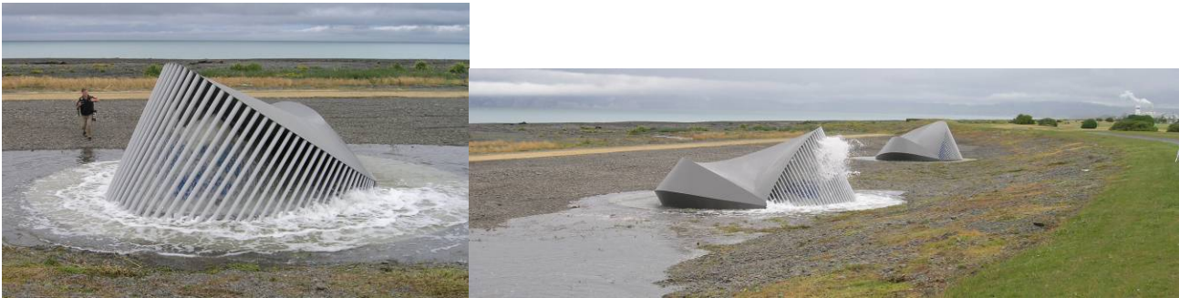
Photograph 6: Main pump start-up – first of three
