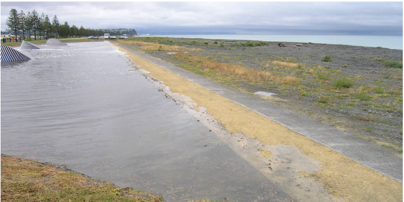
Photograph 7: Full operation – sill about to overflow to beach
