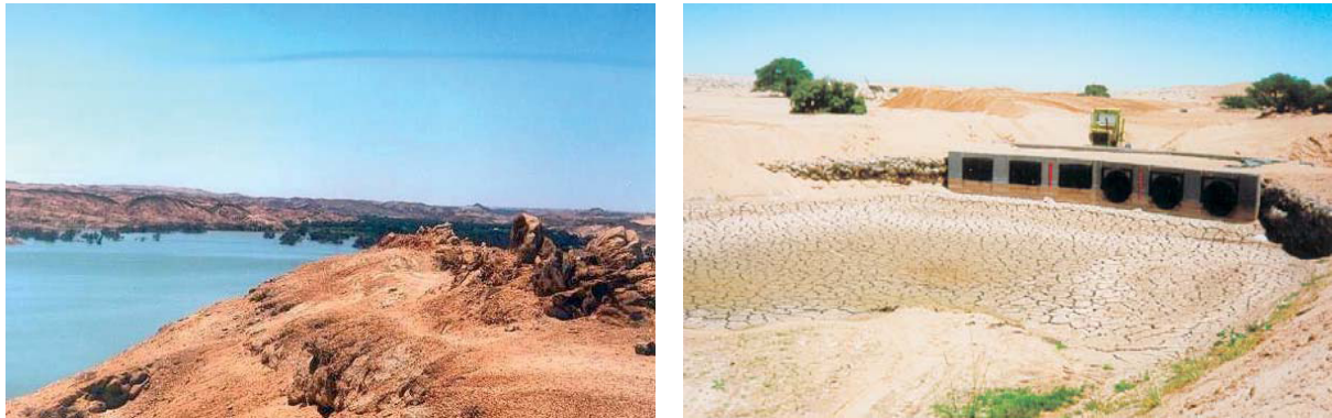
Figure 5. Photographs of Omaruru River Delta Artificial Recharge Scheme.
