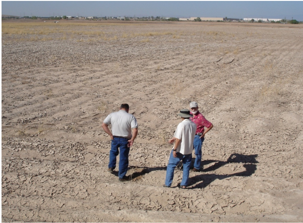
Figure 3. Recharge basin at the NAUSP recharge facility (note the desiccated clogging layer).
