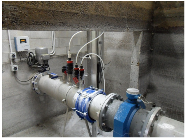
Photograph 4: Converted settling tank
