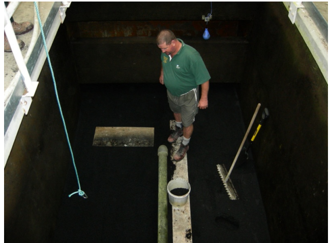
Photograph 5: Filter media installation.
