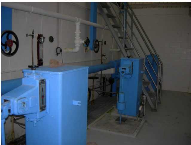
Photograph 6: Old filter gallery
