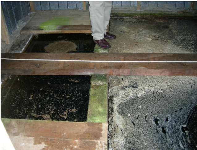
Photograph 3: Old leaf settling tank
