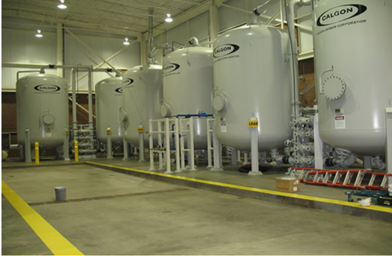
Photograph 2: Biological Activated Carbon Filters utilising pressure vessels
