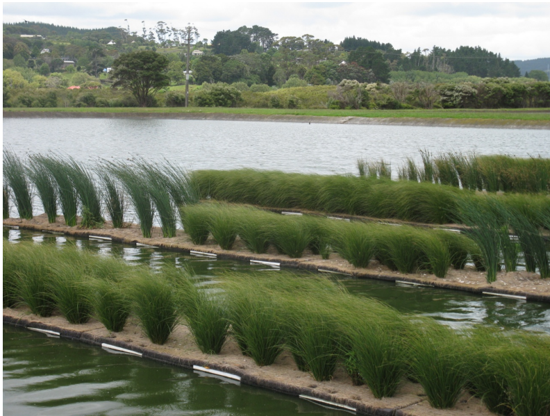
Photograph 1: Different Plant Species Trialed at the Helensville Wastewater Treatment Plant
