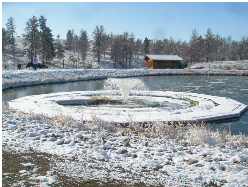
Photograph 7: Floating island after installation, November 2009
