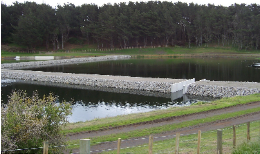
Photograph 7: Completed internal dividing bunds
