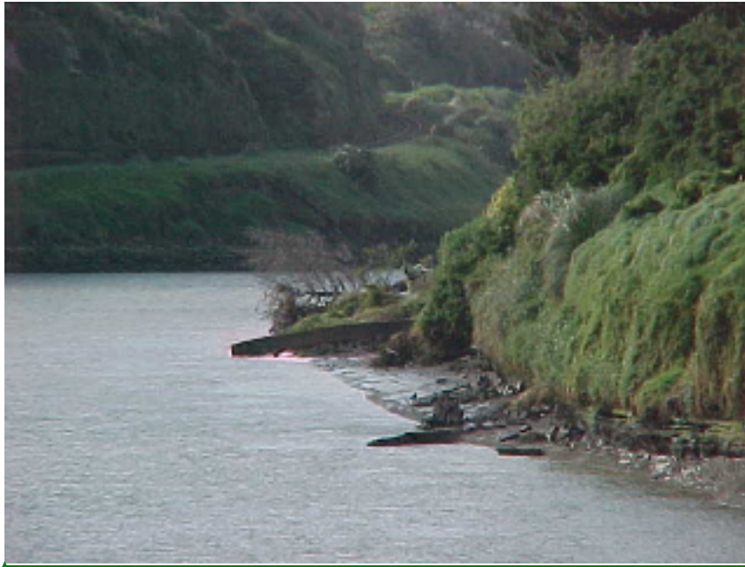
Photograph 3: WWTP outfall to Patea River at low tide, viewed from upstream (note pink Rhodamine WT dye from mixing and dilution experiment near bank from cracks in outfall pipe)
