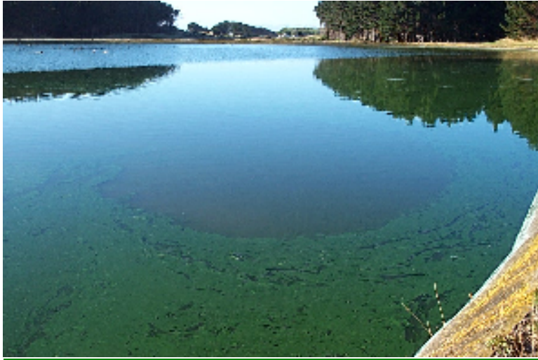
Photograph 1: Oxidation pond before the upgrade, showing inflow welling up in centre of photo
