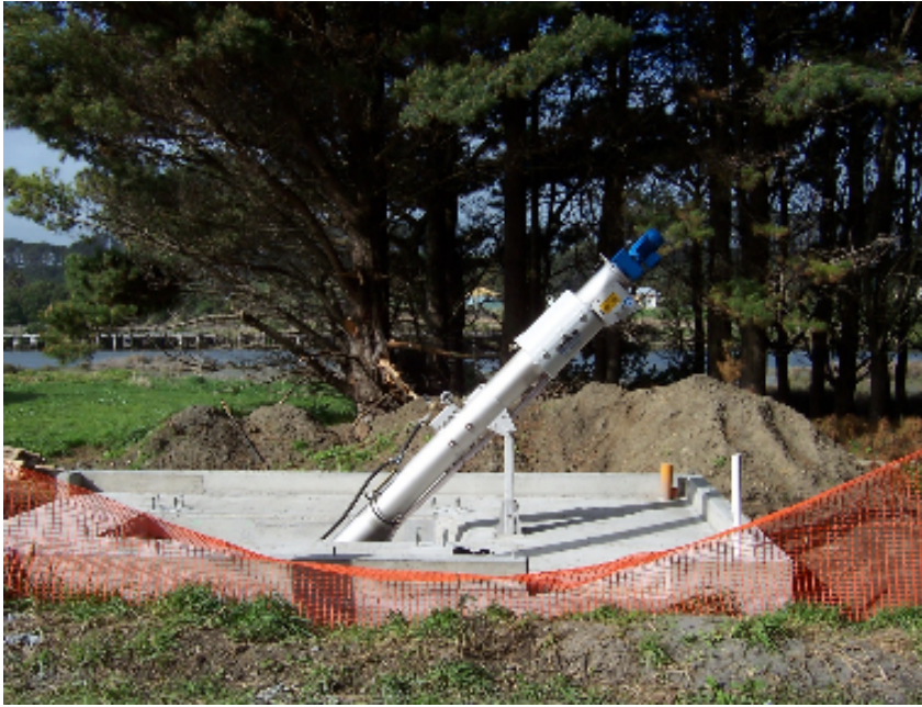
Photograph 4: Rotary auger screen (during construction)
