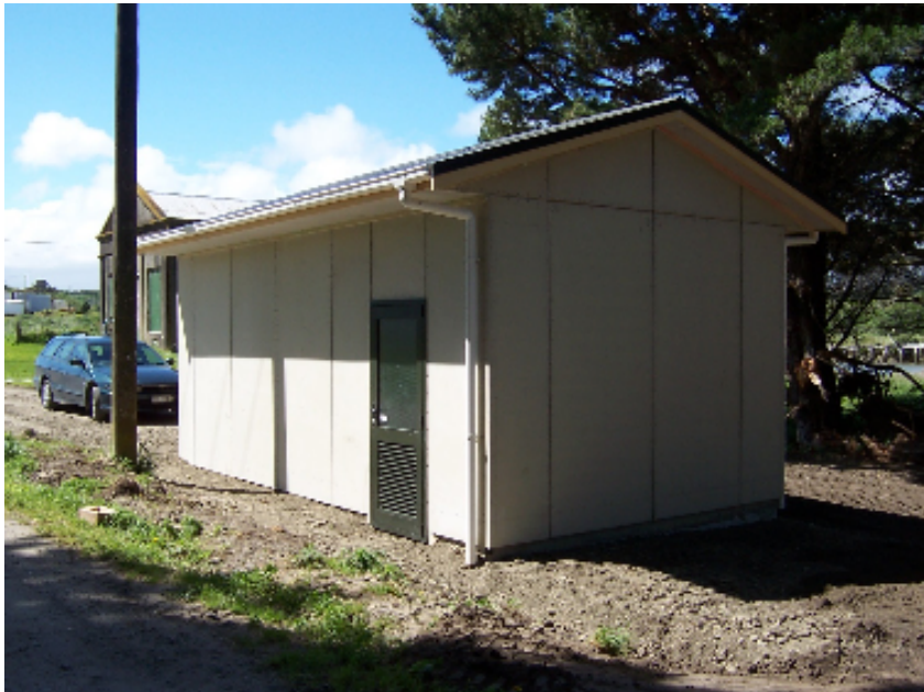
Photograph 5: Shed housing the rotary auger screen
