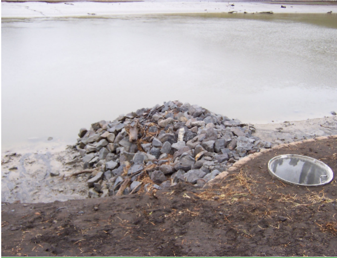
Photograph 8: In-bank rock diffuser
