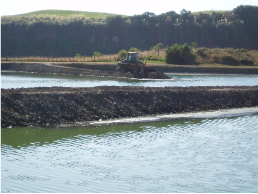
Photograph 6: End-dumping rock to create internal bunds
