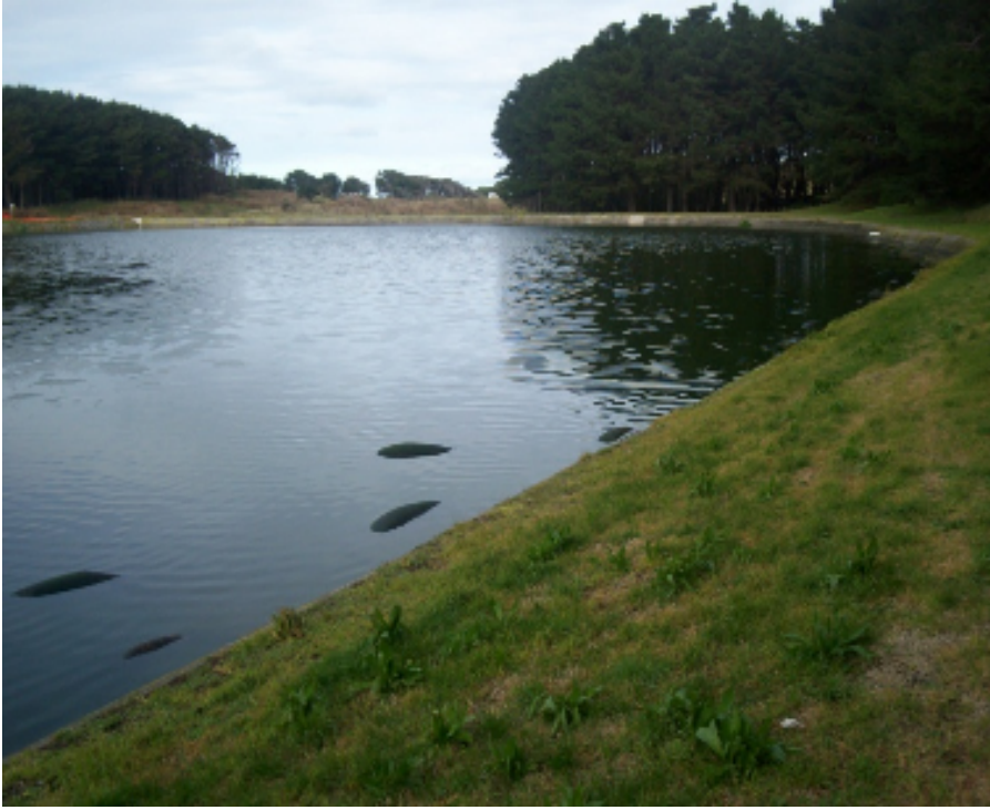
Photograph 9: Pond liner ballooning to surface, buoyed by biogas
