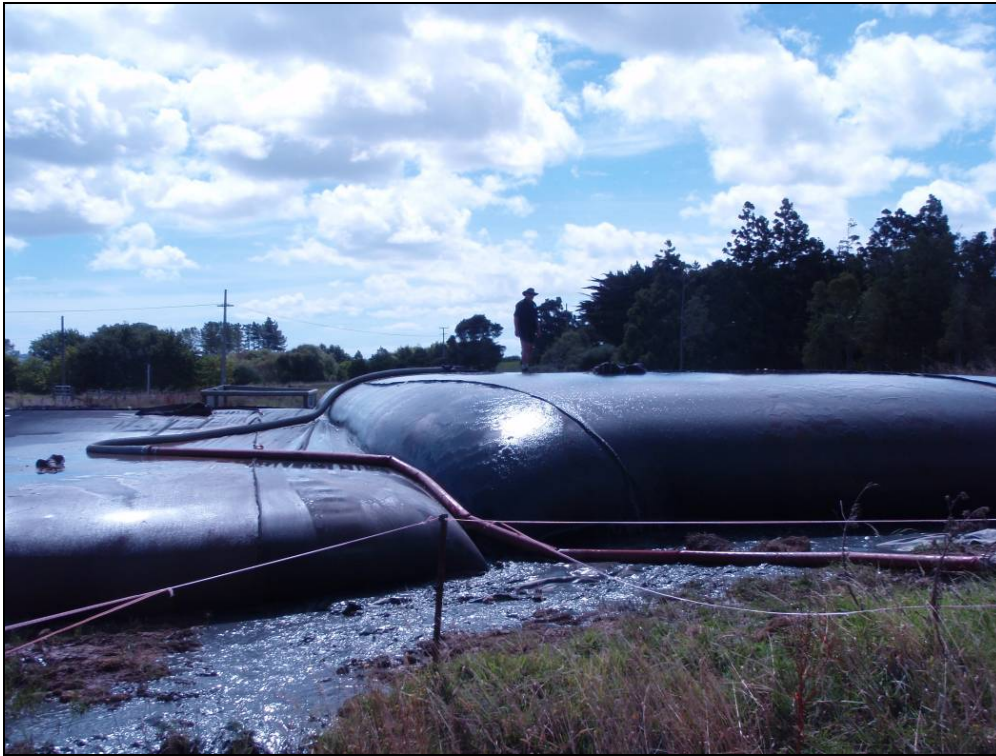
Photograph 9: Geo-Textile Filter Bags being filed.
