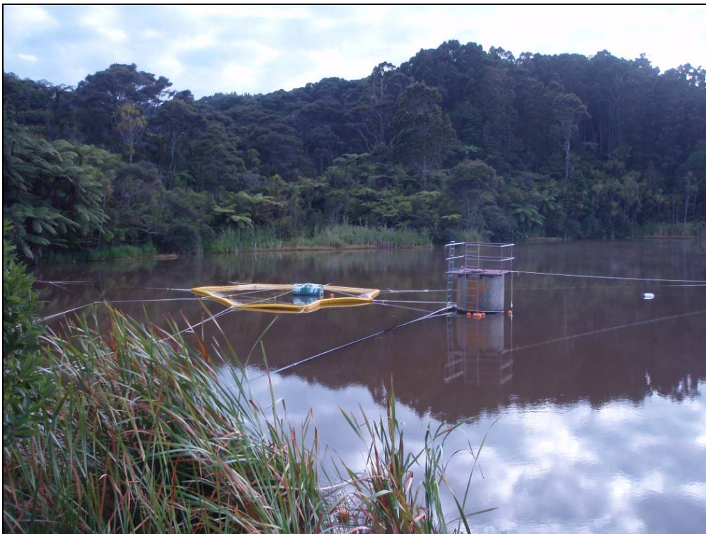
Photograph 5: Floating Filter Cloth around Intake.
