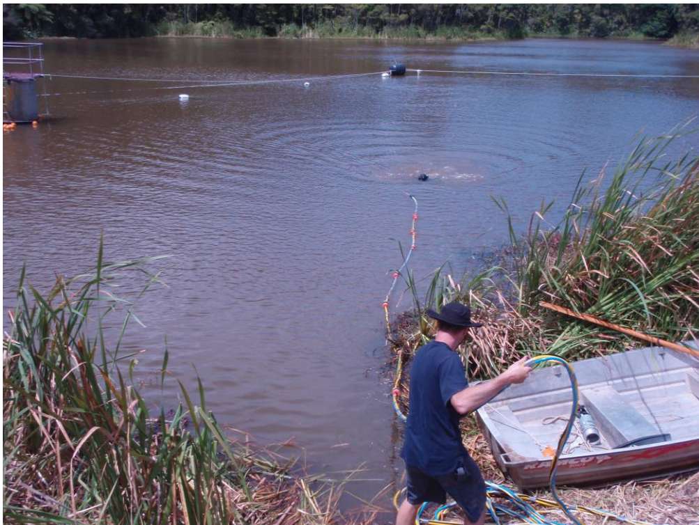
Photograph 7: Diver on Surface Supply Swimming to Dredge Face.
