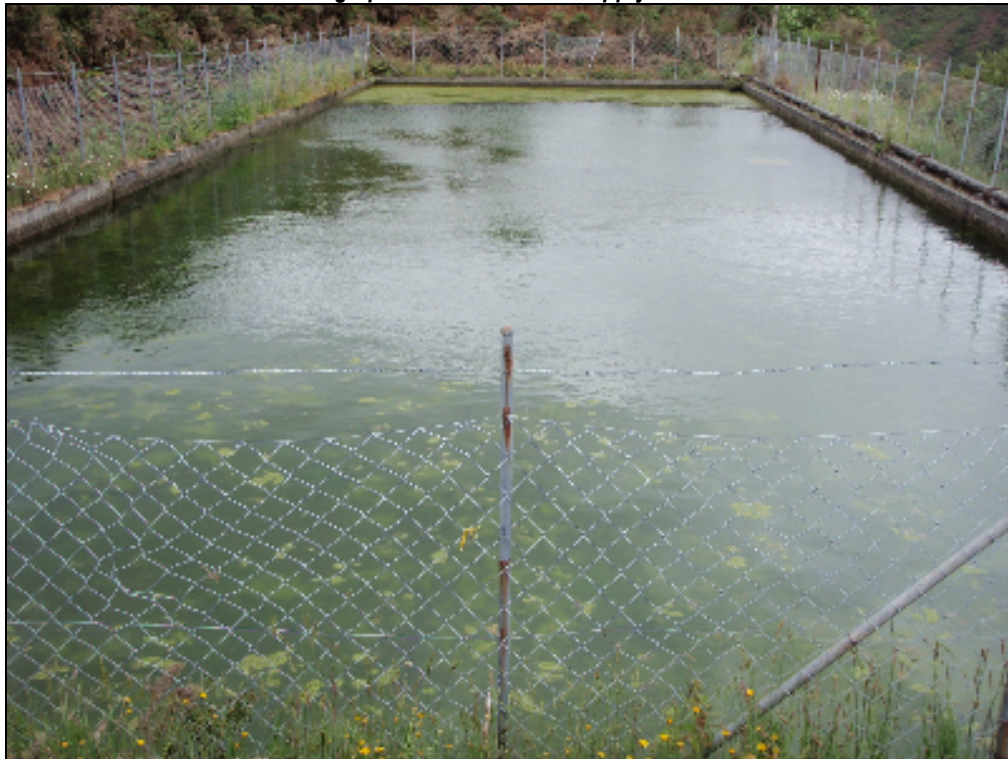
Photograph 2: Reefton water supply reservoir
