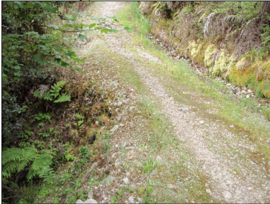
Photograph 3: Section of access track to reservoir
