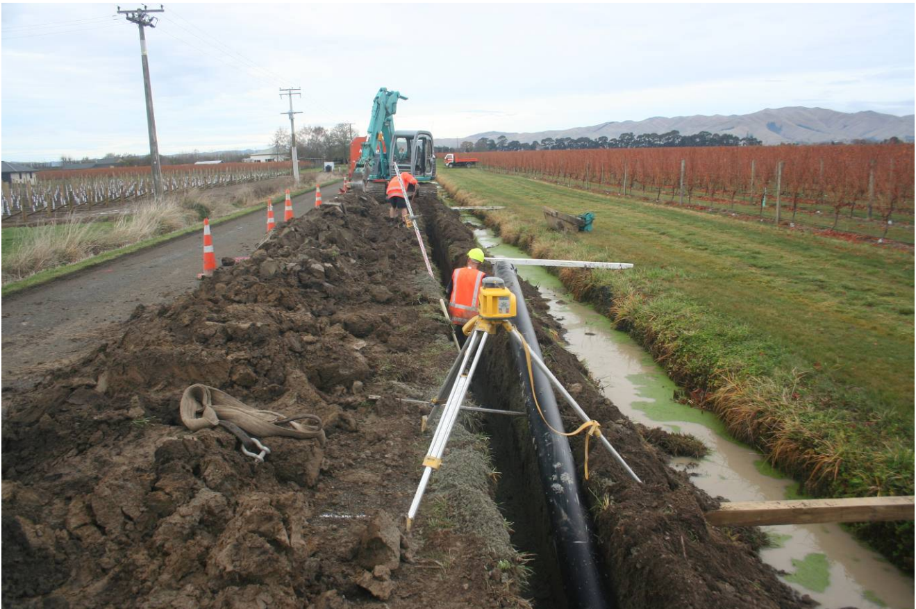
Photograph 4: Laying PE Pipe Adjacent to Open Drains with High Groundwater
