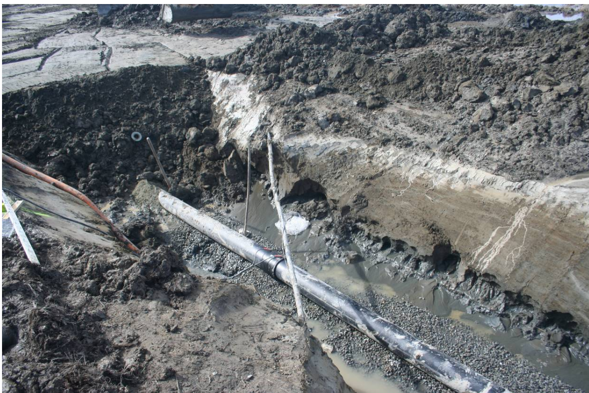
Photograph 1: Running Sand in a Trench During Installation
