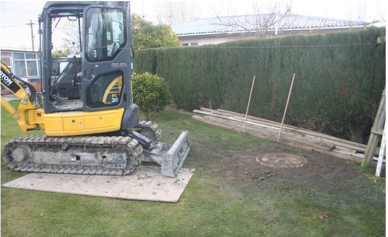
Photograph 3: Top of Grinder Unit After Reinstatement
