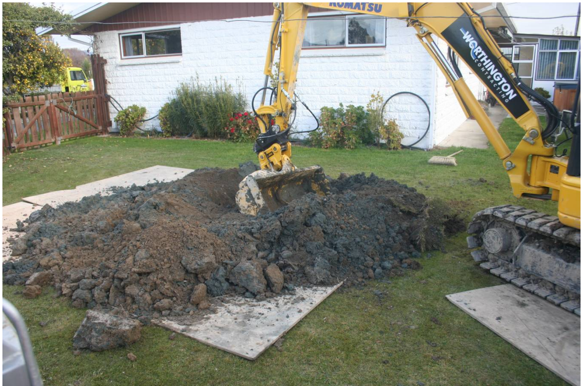
Photograph 2: Minimising Impact on Private Property by Using Boards
