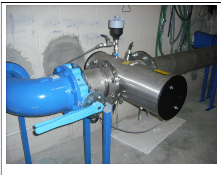
Photographs 2 and 3: Frederick St supplementary supply UV chamber and control interface
