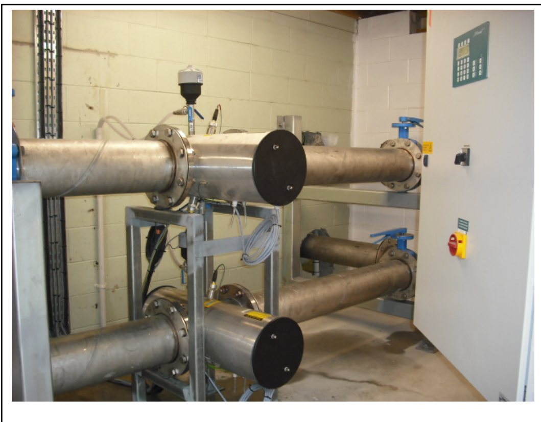
Photographs 2 and 3: Frederick St supplementary supply UV chamber and control interface
