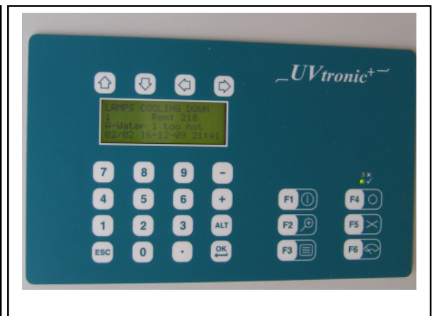
Photographs 2 and 3: Frederick St supplementary supply UV chamber and control interface
