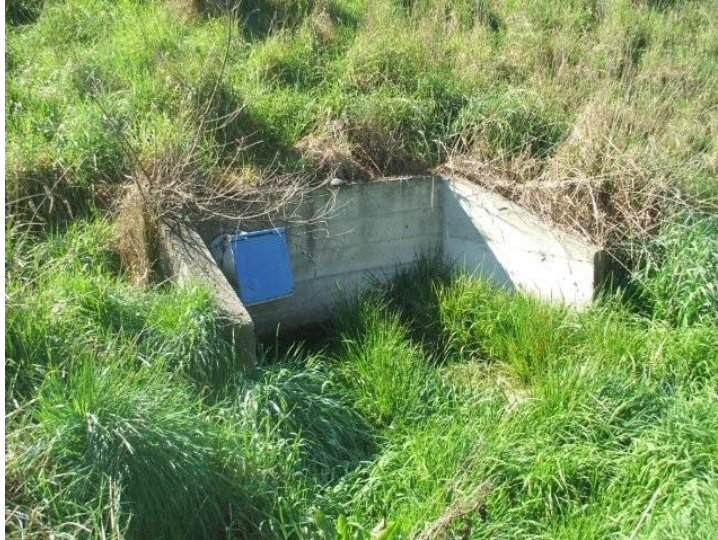
Photograph 3: Pump Station Overflow
