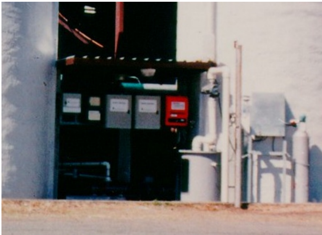
Photograph 1: Earliest WS remote monitored pilot plant set up outside Brisbane and monitored from Dunedin. Data Logger is the box on the left. The others contain an SLC500 PLC, VFD and other control equipment. It was not practical at the time to have both logger and PLC remote connected.
