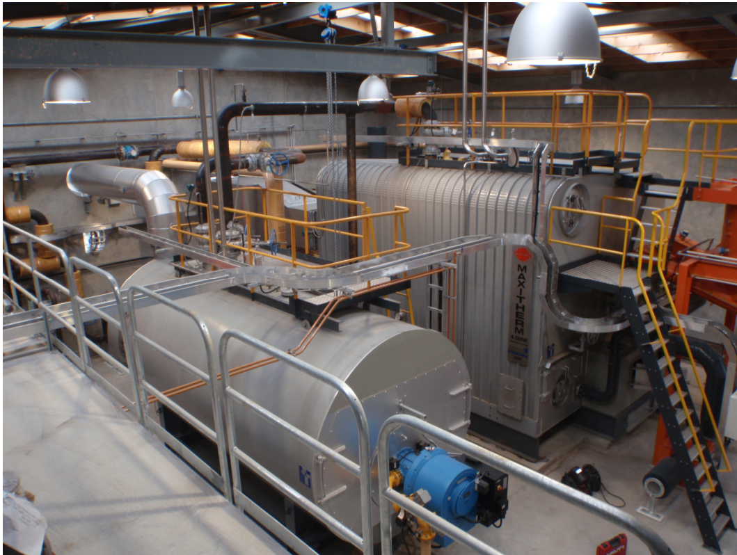
Photograph 1: Biosolids Drying Plant Energy Centre
