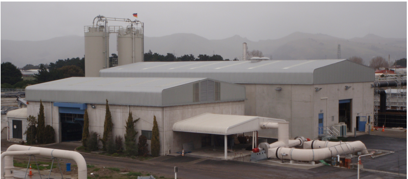
Photograph 3: Christchurch Biosolids Drying Building (Dewatering Building in Front)
