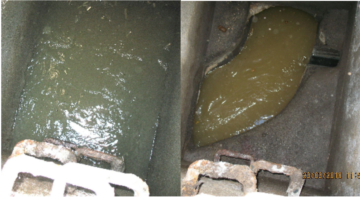
Photographs 3 & 4: Before (10:50am) and after (11:58am) at manhole 2819795, 450m upstream
