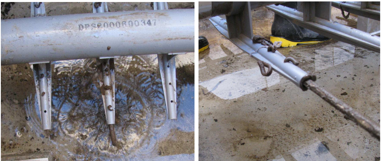
Photograph 7: Coarse Bubble Aeration Diffuser Cleaning [Te Aroha WWTP]
