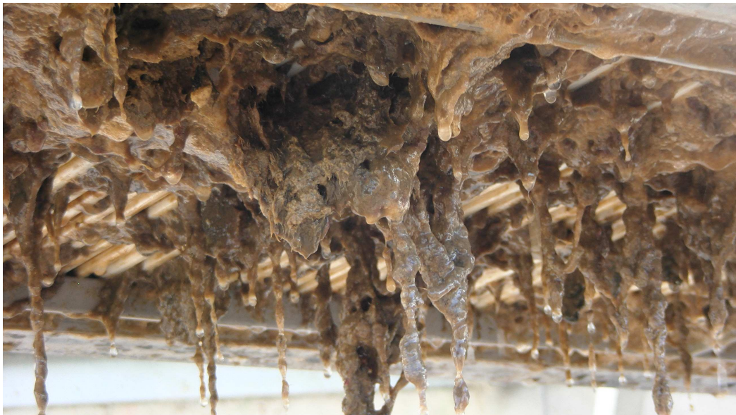
Photograph 4: Example of lint/hair agglomeration at the base of a membrane module (Turangi WWTP)
