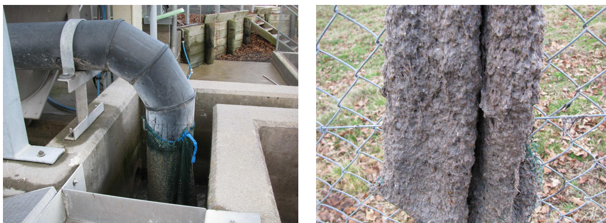
Photograph 5: Crude additional screening provided at the Tirau WWTP to reduce quantities of ling entering process
