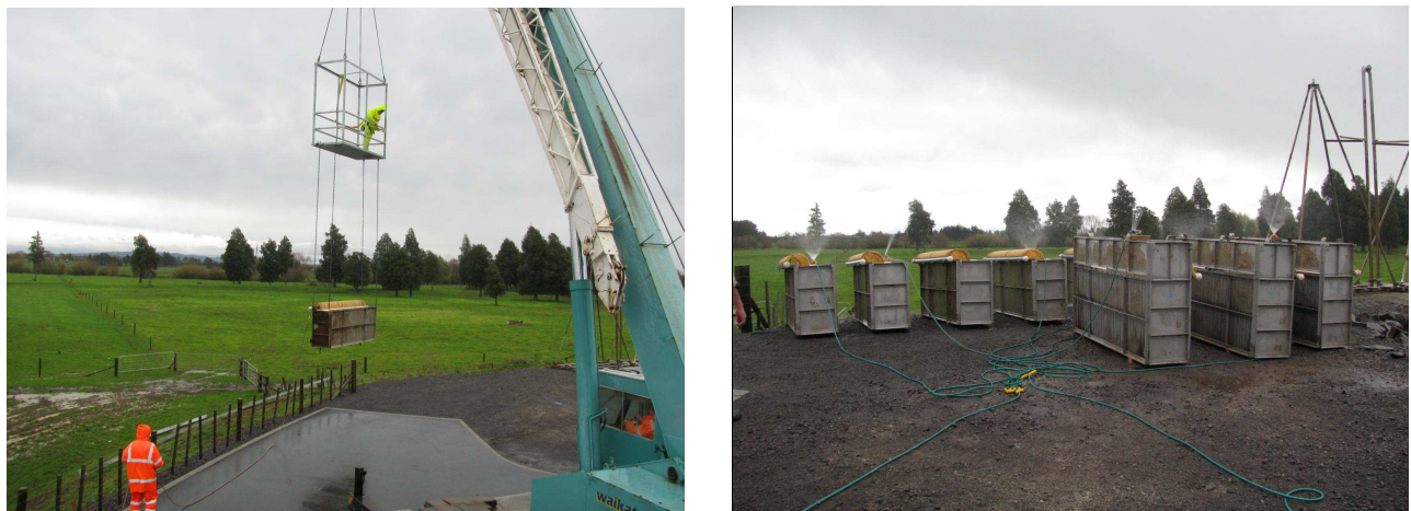
Photograph 8: Membrane Module Removal and Temporary Storage
