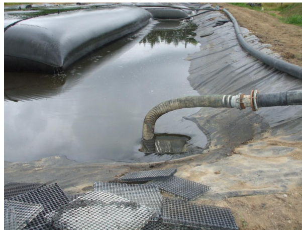
Photograph 2: Pumped Return to Oxidation Ponds
