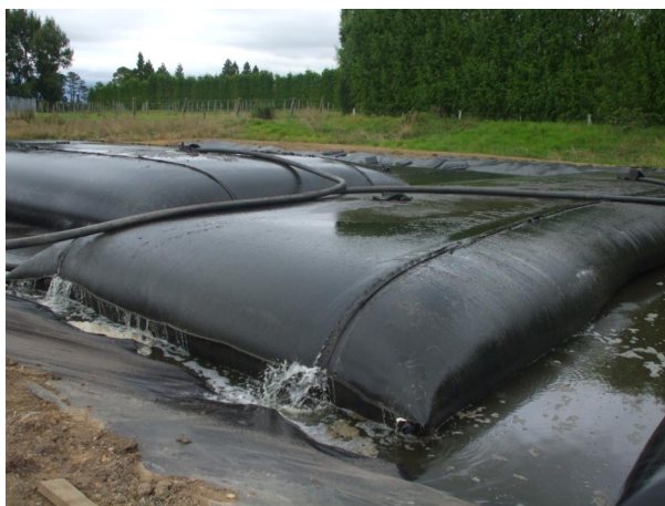
Photograph 1: Early Stages of Dewatering
