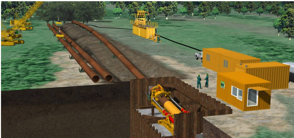
Figure 4: Pipeline sections thrust by the Pipe Thruster.
