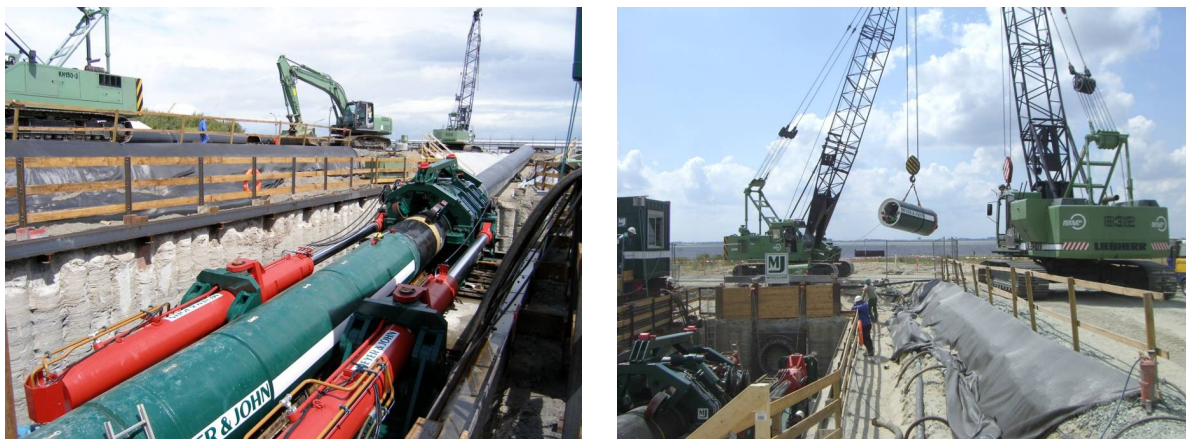
Figure 11: Second Direct Pipe®-project in Emden, Northern Germany. Jobsite installation.
