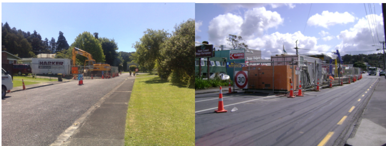
Photographs 4 and 5: Jacking Shaft Sites in Suburban Areas
