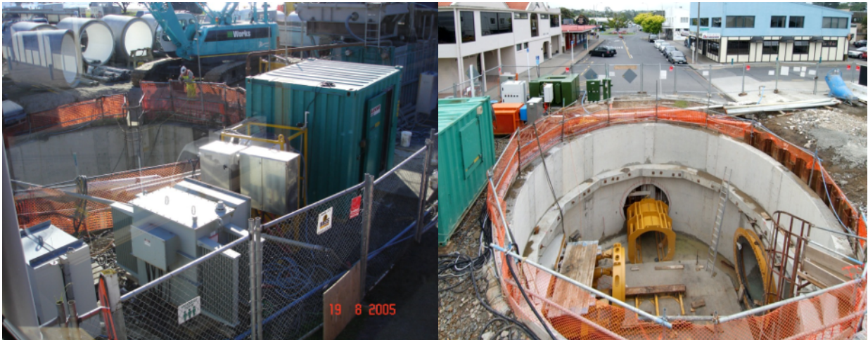
Photographs 7 & 8: Jacking shaft site on micro tunnelling project in Browns Bay
