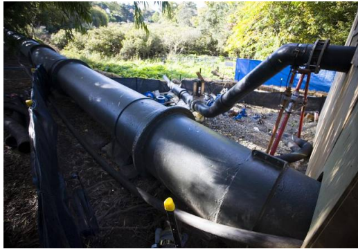
Figure 22 bypass pipe setup at grit chamber
