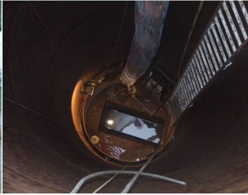
Figure 30 Sewer crown opened up
