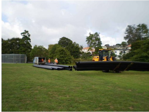
Figure 22 bypass pipe setup at grit chamber
