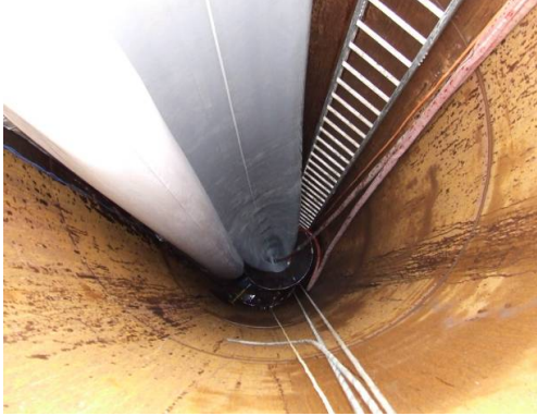
Figure 39 Liner running to inversion chute
