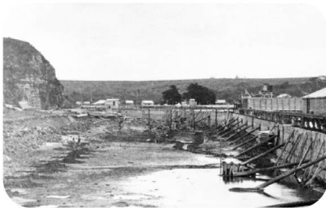
Figure 6 – Orakei main storage tanks
