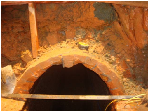
Figure 41 Branch 1 sewer at shaft base, before lining
