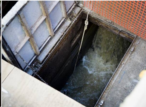
Figure 23 Flow entering grit chamber
