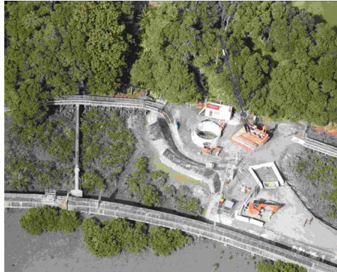
Figure 18 MH01 location- in Project Hobson site
