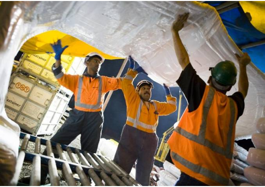
Figure 33 Liner preparation for impregnation
