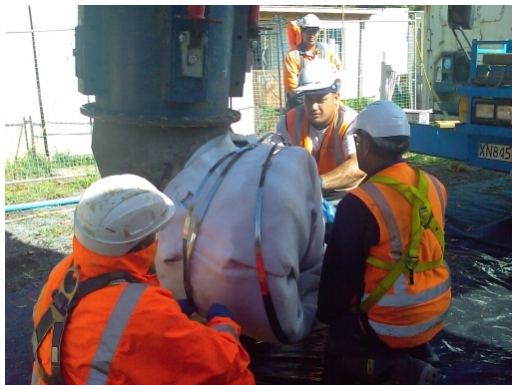
Figure 37 Liner attachment to steel chute
