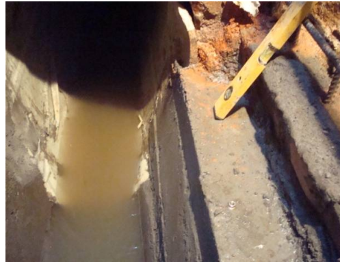
Figure 42 Shaft base reinstatement after lining
