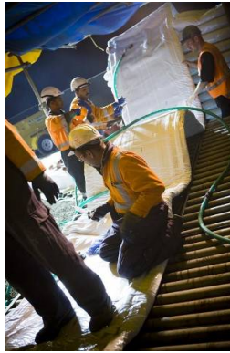
Figure 34 Liner vacuuming
