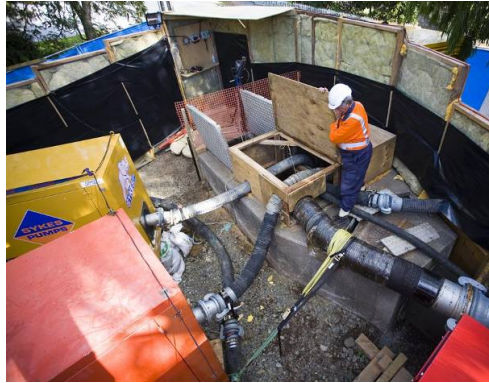
Figure 23 Flow entering grit chamber
