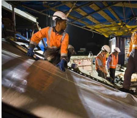
Figure 36 Liner impregnation
