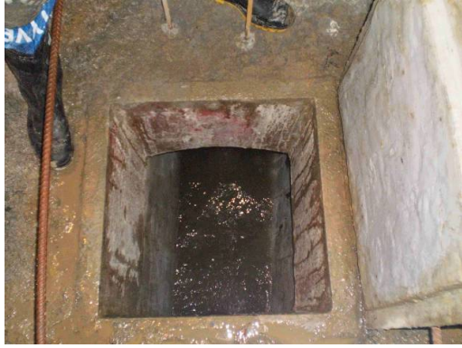
Figure 43 Shaft base, with resin lining
