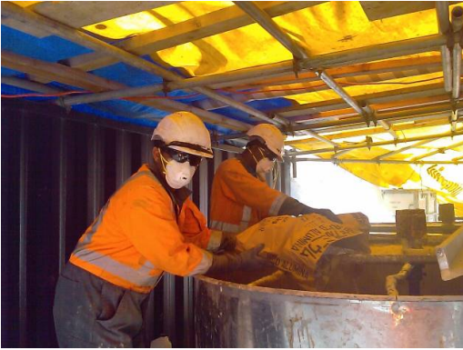
Figure 35 Resin mixing
