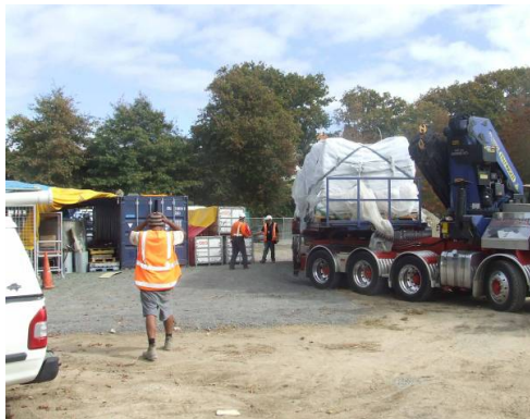
Figure 31 Liner arrival at site
