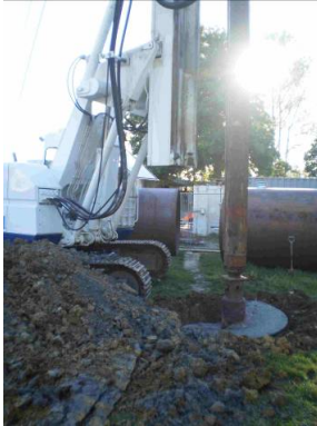
Figure 27 Auger drilling temporary shaft
