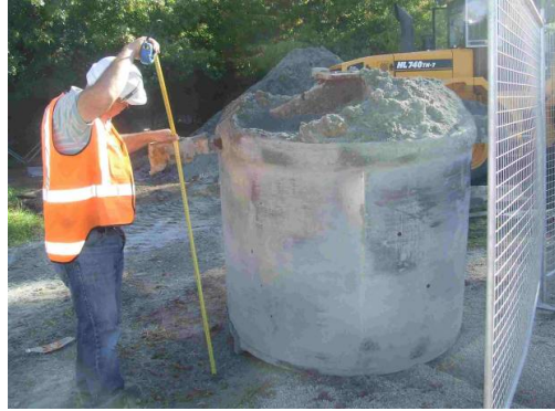
Figure 28 “apple coring” head for drilling
