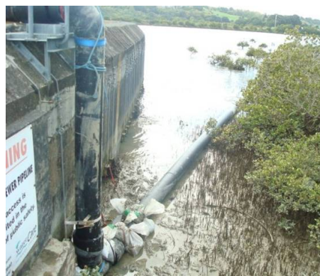
Figure 25 Bypass pipe arriving at Orakei Main
