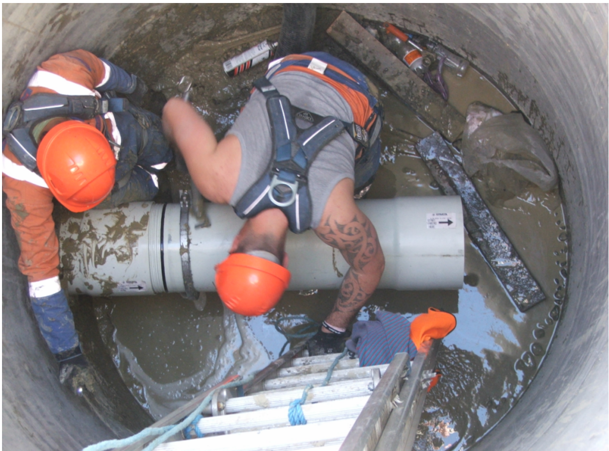
Photograph 4: Iona mews; Assembling 1 metre Restrain™ inside the 1800 dia manhole at a depth of 5.7 metres
