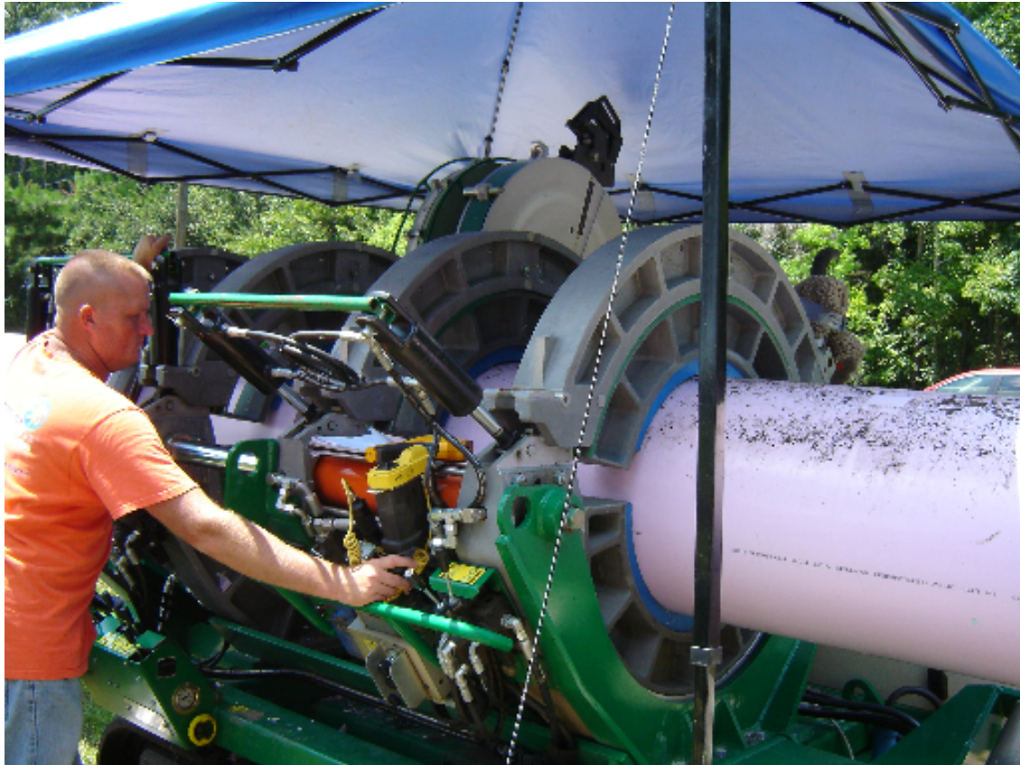
Photograph 2: Fusion welding of FPVC™ pipe.
