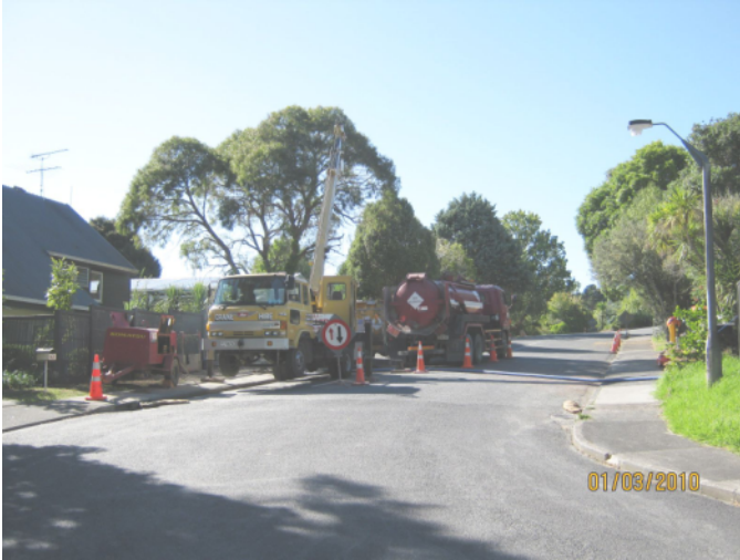
Picture 11 (left): Mud removal from manhole
