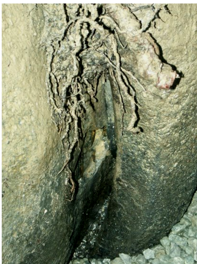
Photograph 5: Detail of joint leak and root intrusion and general view of area
