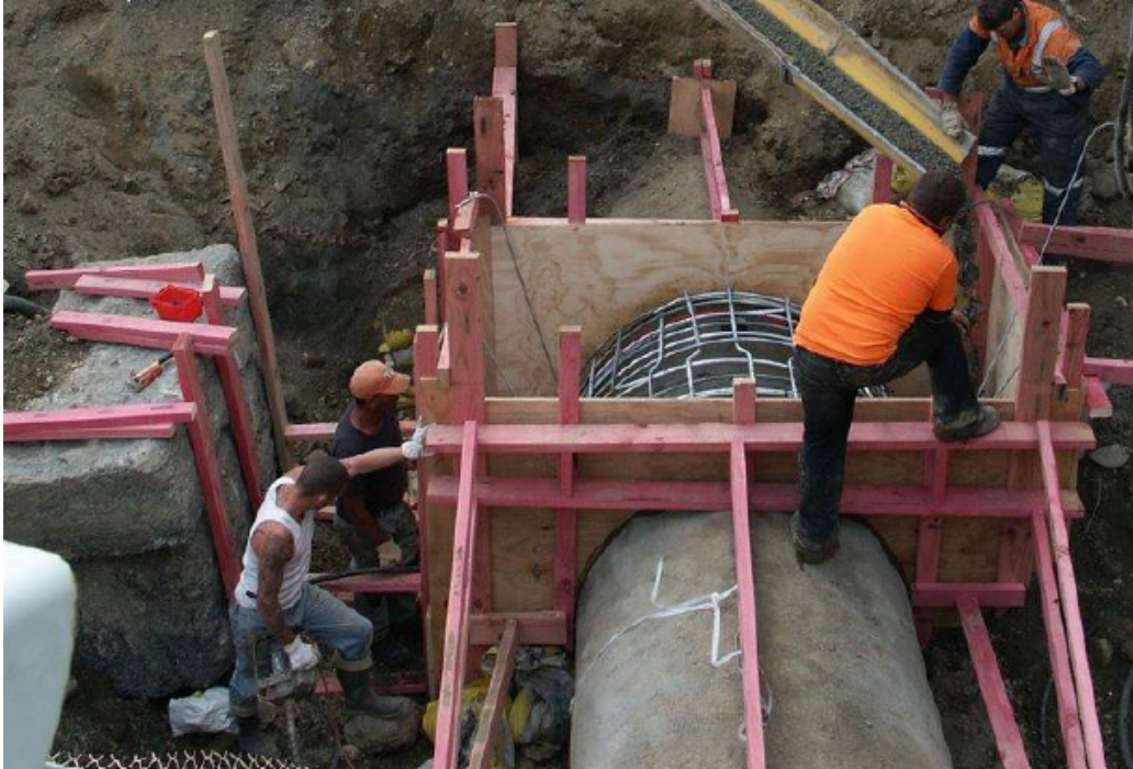
Photograph 4: Concrete bandage being poured at the first joint leak repair
