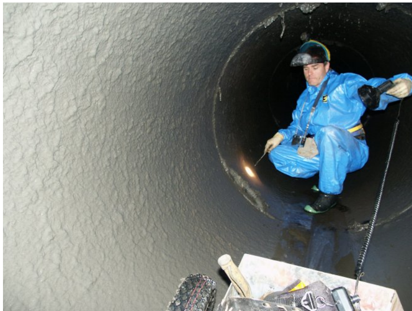
Photograph 2: Internal condition inspection 2004
