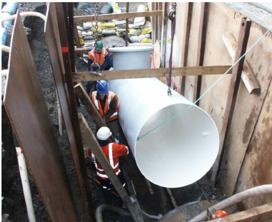
Photograph 7: Lowering the final steel section in for slip-lining
