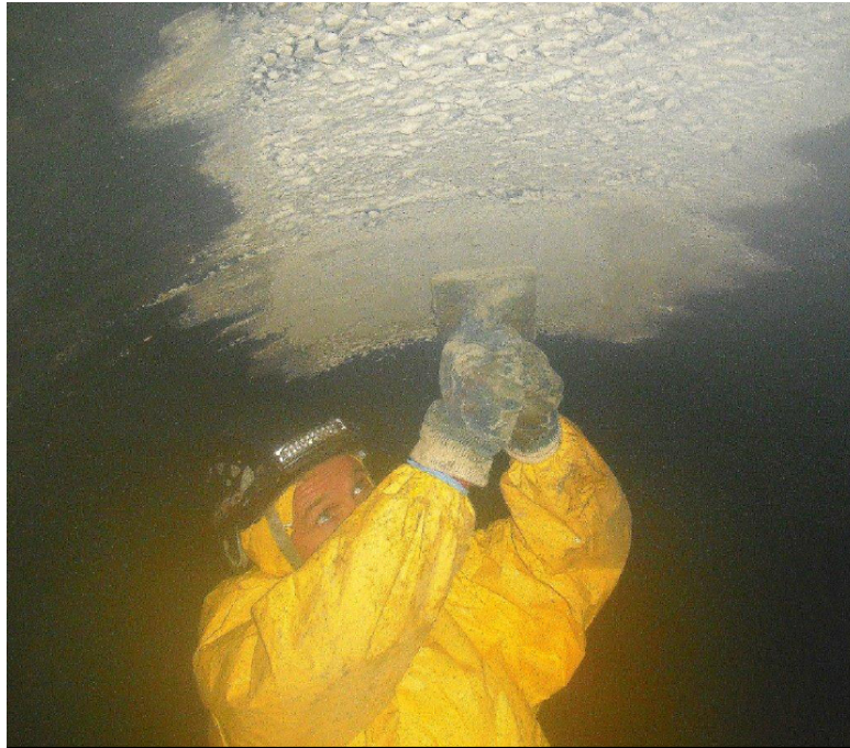
Photograph 9: Repair of pipe soffit prior to placing internal AMEX seal
