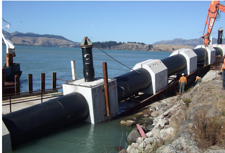
Figure 5 – Launching diffuser section on slipway at Lyttelton CMA
