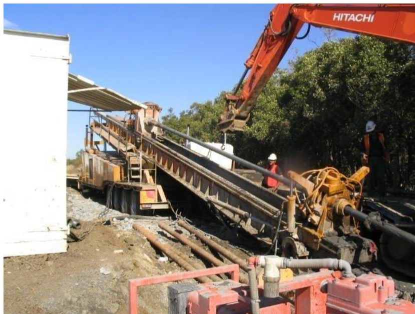
Photograph 5: HDD drill rig on the south side of Brisbane River.
