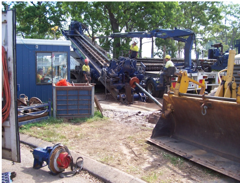
Photograph 7: HDD drill rig at Victoria Point, drilling towards Coochiemudlo Island.
