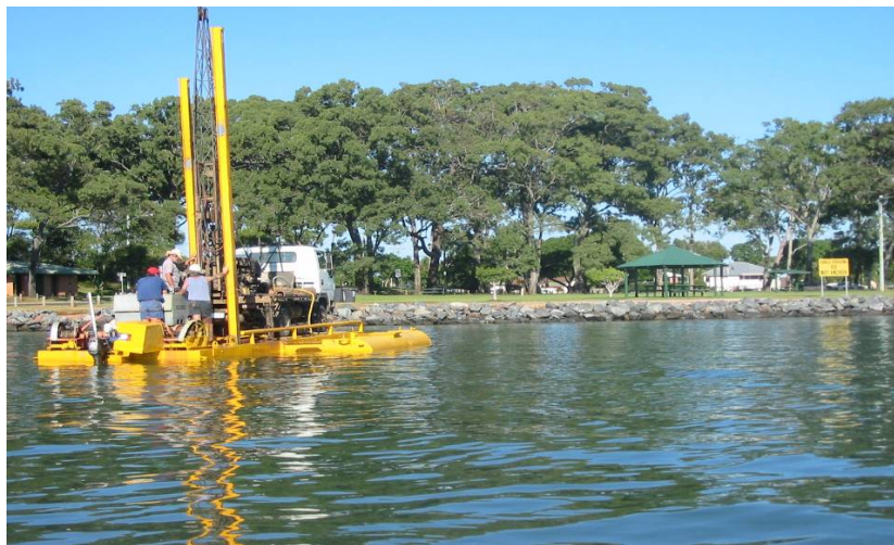
Photograph 3: Moreton Bay geotechnical drilling off Victoria Point.
